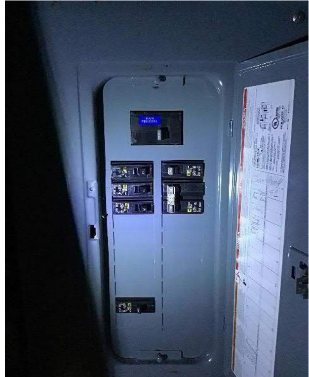
View of breaker box #2 circuit breakers located in the basement facing Southwest.
