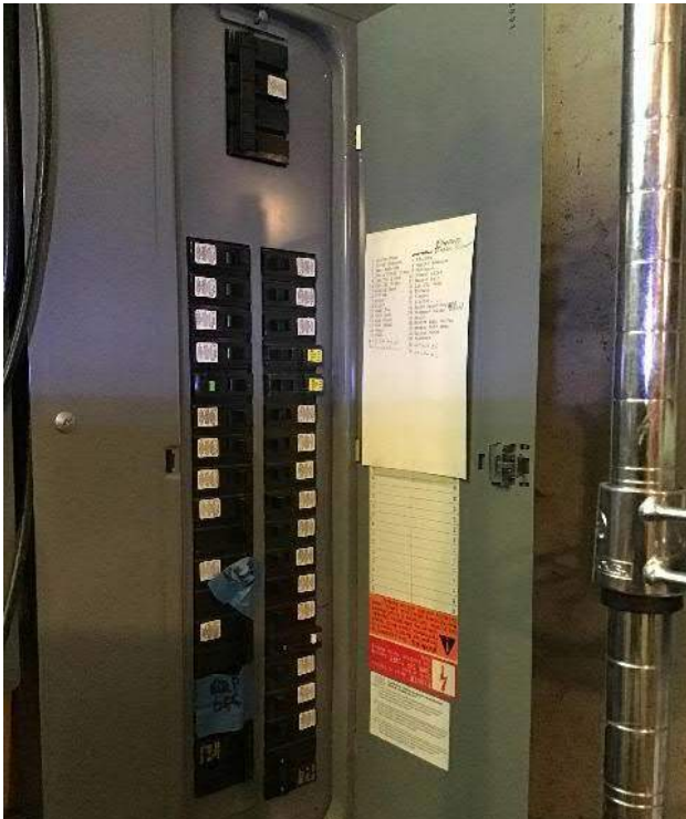
View of breaker box #2 front panel open.
