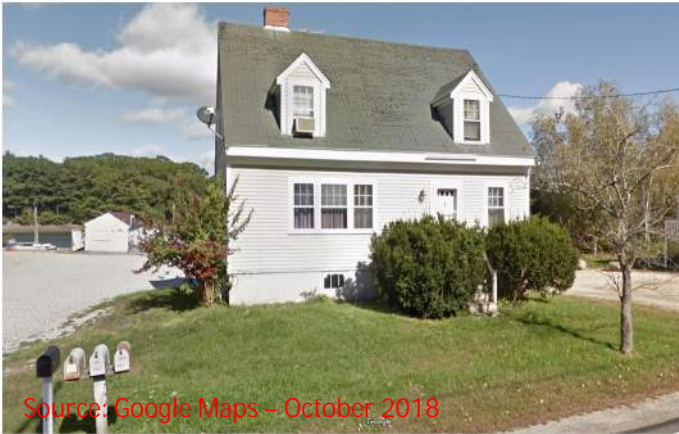
View of 187 Wentworth House Road from the road with gravel driveways on either side, facing North.
