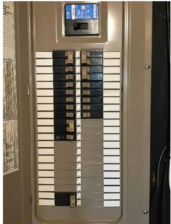
View of breaker box #1 (Eaton) circuit breakers facing Southwest.
