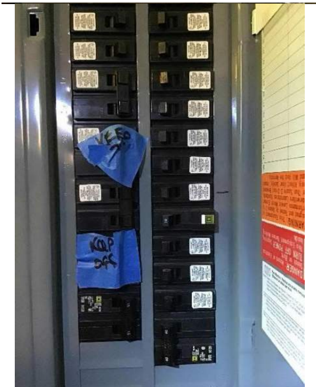
Continued view of breaker box #2 circuit breakers.
