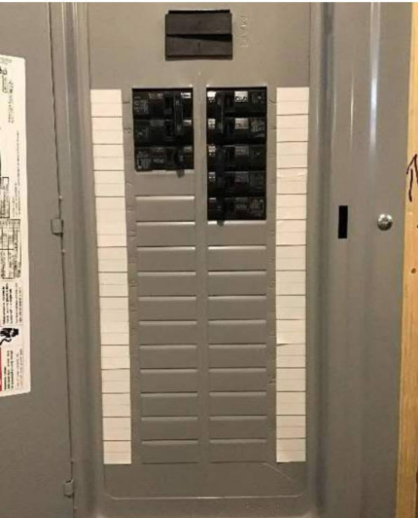
View of breaker box #2 circuit breakers.
