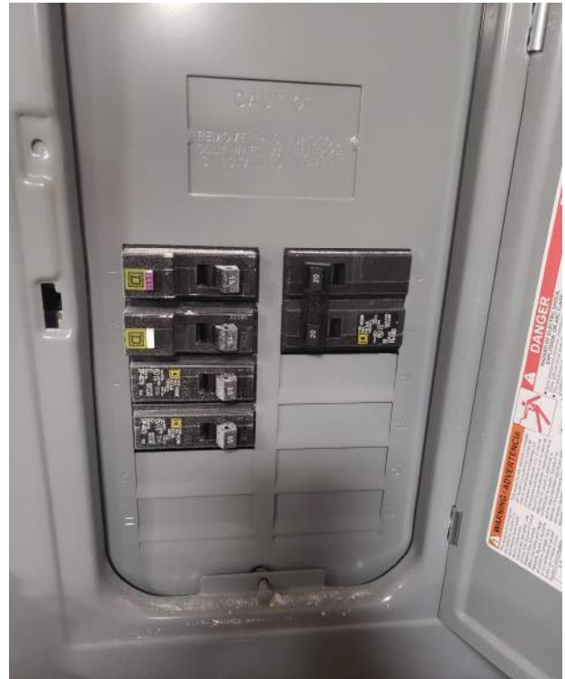
View of breaker box #2 circuit breakers.
