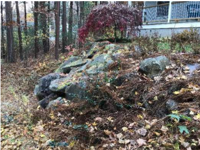
View of second retaining wall in front of the house facing South.
