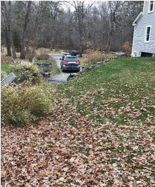
View of driveway facing Walker Bungalow Road and retaining wall facing Northeast.
