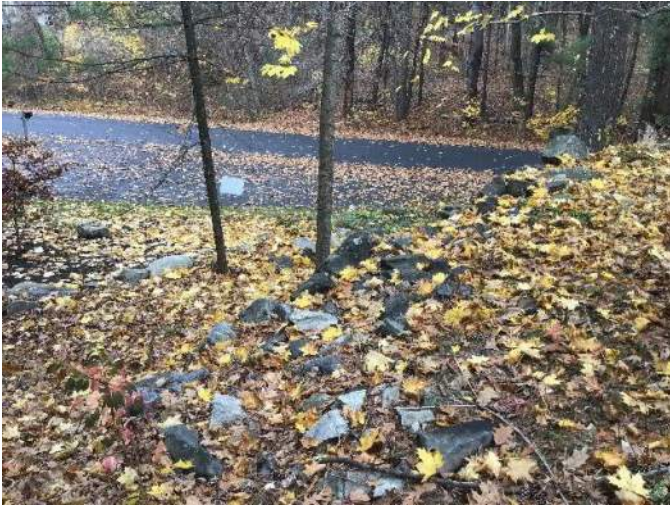
View from the top of the retaining wall down towards the road facing Northeast.
