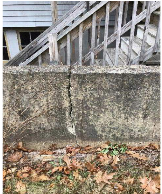
View of large crack and spalling in the concrete retaining wall facing Southwest.
