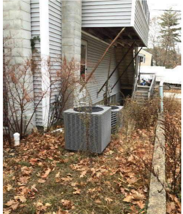
View of AC units and concrete retaining wall along the rear of the building facing Northwest.
