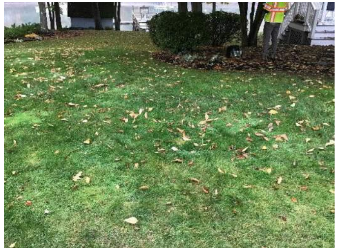
View of approximate location of buried septic tank in the East yard, facing Southwest.
