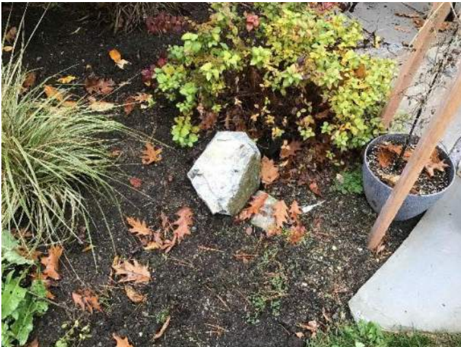
View of approximate septic tank cap location within the shrubs facing Northwest.
