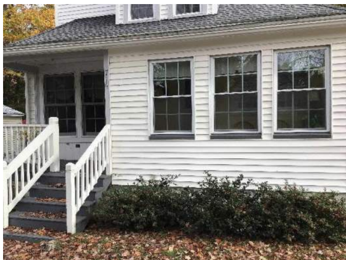
View of 714 Avenue from the front yard facing Northeast.
