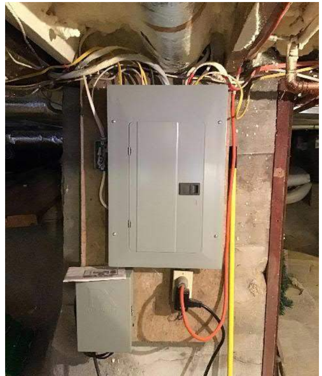
View of breaker box #1 located in the basement facing West.
