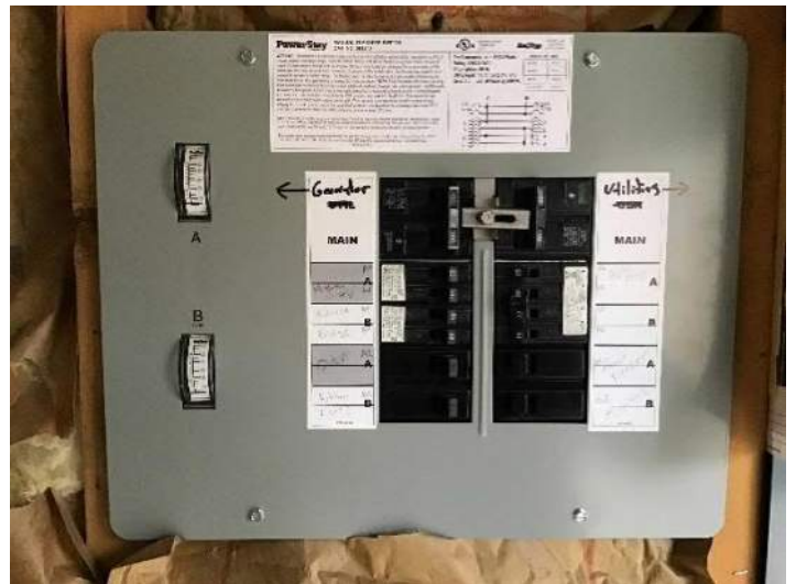
View of manual transfer switch front panel and schedule adjacent to the breaker switches.
