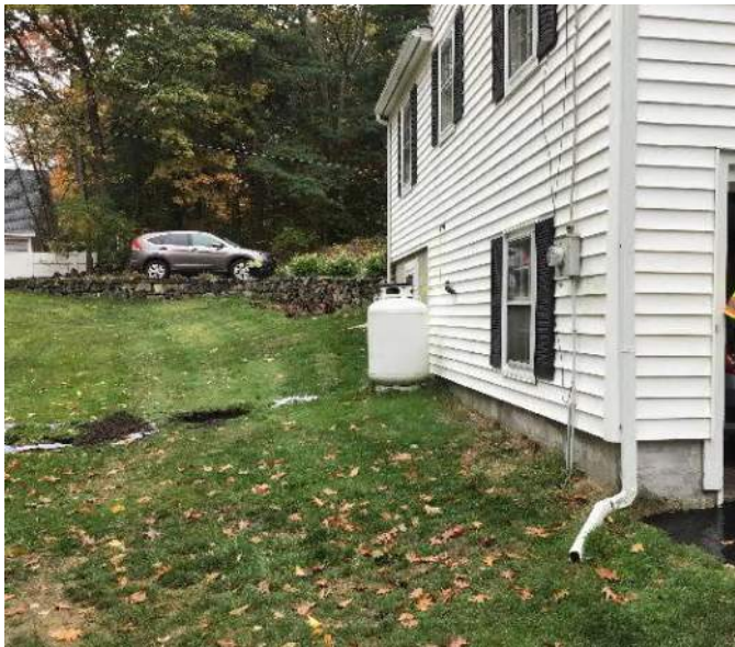
View of the first septic tank and lateral exit with turf removed, located on the Southeast side of the house facing Southwest.
