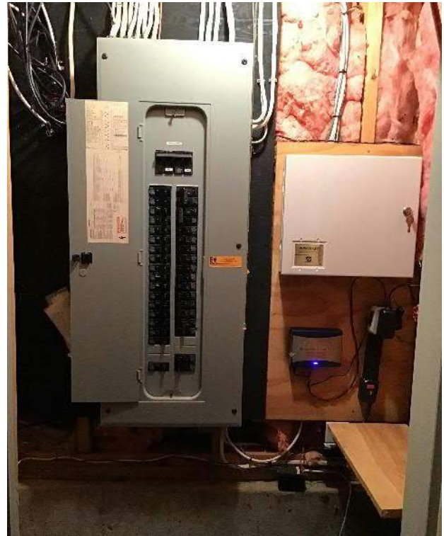
View of the breaker box and surrounding wall space located in a basement closet, facing Northeast.
