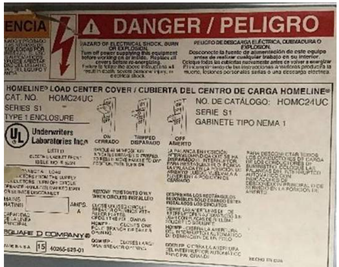
View of breaker box model information and specifications.
