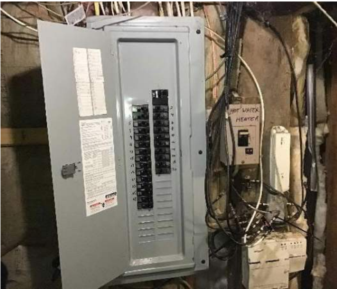
View of the breaker box and surrounding wall space located in the crawlspace facing West.
