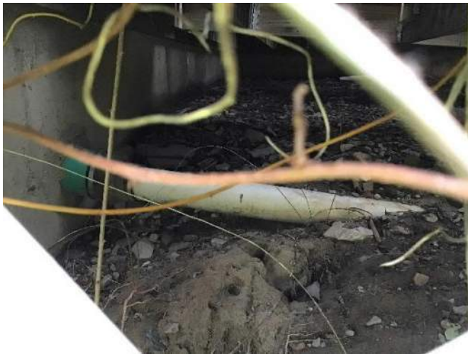
View of exposed PVC sewer lateral exiting the foundation facing Southwest.
