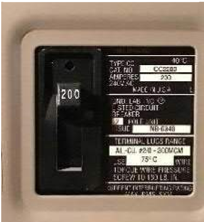
View of the main breaker switch and breaker box model information.
