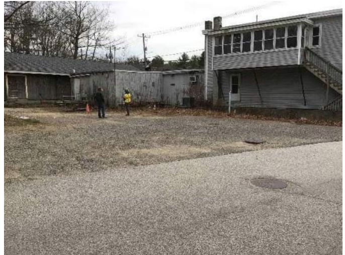
View of the rear gravel parking lot and approximate location of buried concrete tanks facing Southwest.
