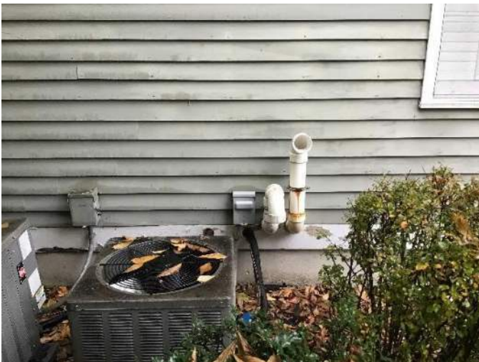
View of approximate location of the buried sewer lateral, facing West.
