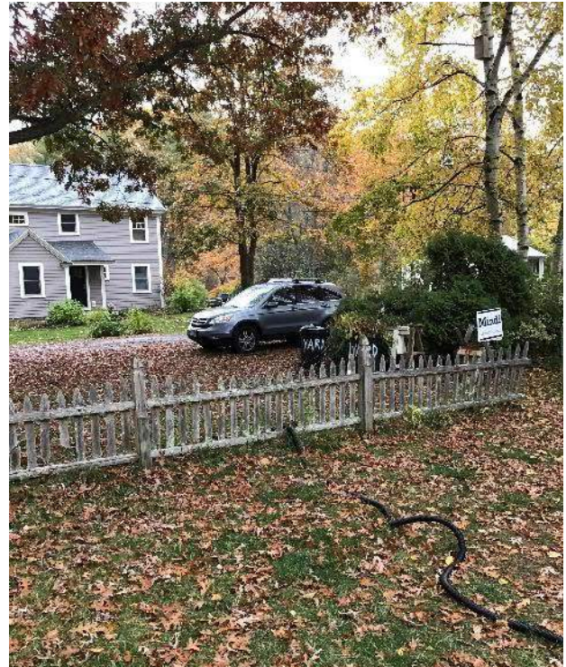
View of wooden fence crossing proposed sewer service path located in the backyard, facing East.
