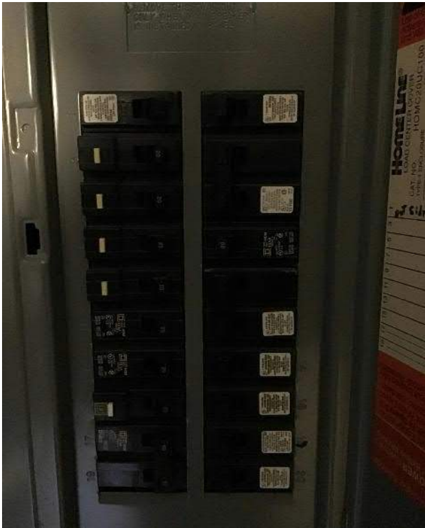
View of breaker box #1 circuit breakers.
