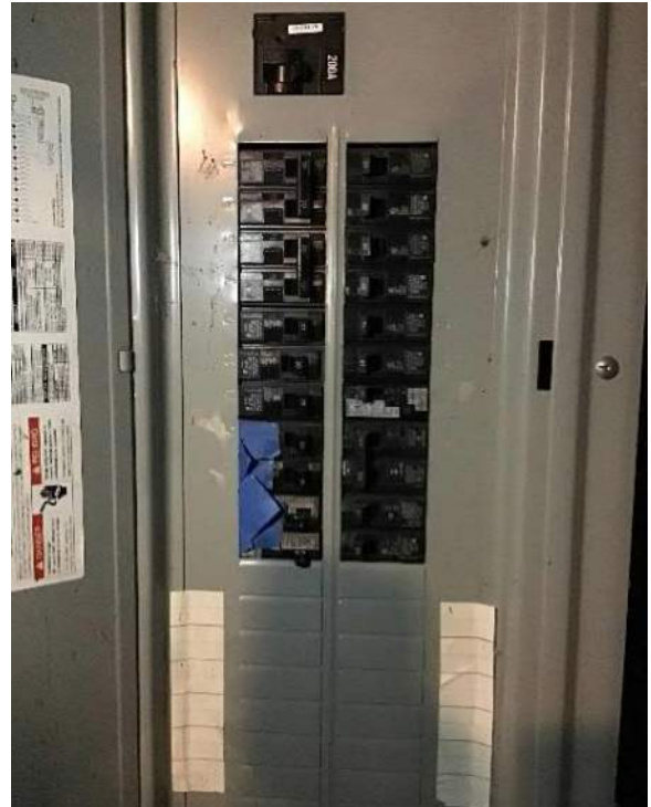
View of Siemens circuit breakers and available slots.
