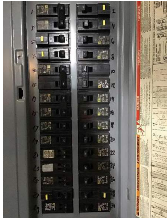
View of breaker box #1 circuit breakers.
