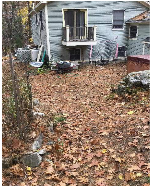
View of approximate location of buried septic tank and pump station, facing Northeast.
