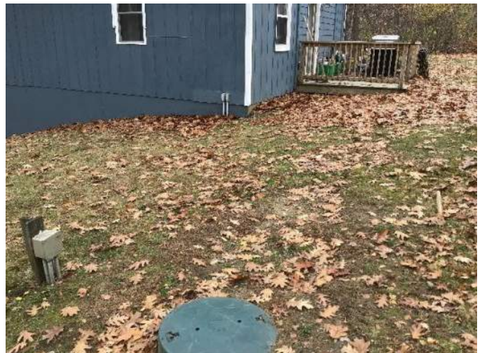
View of underground electrical service and approximate buried sewer lateral location to the house facing Southwest.
