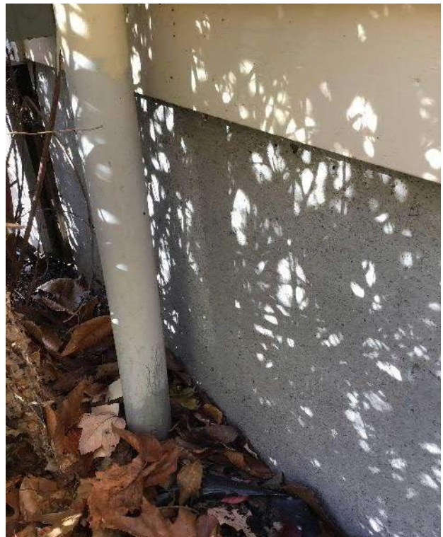
View of electrical conduit routed from the basement on the Southeast side of the house, facing West.
