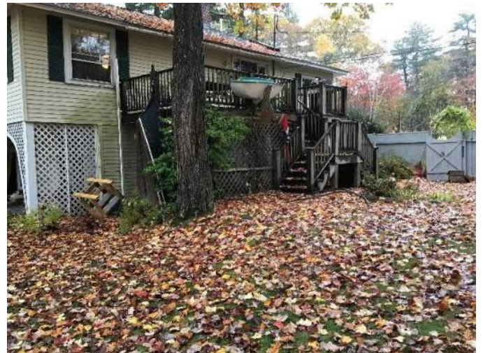
View of large tree and wooden deck and fence on the West side of the house facing Southeast.
