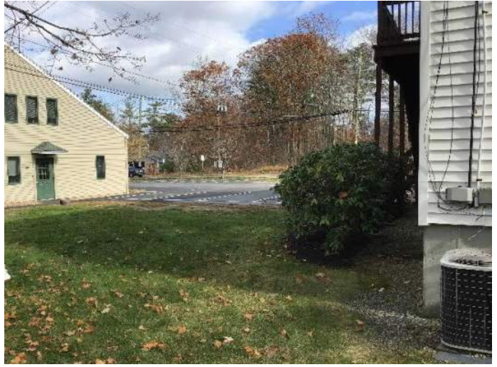
View of the Northwest corner and looking towards the parking lot connected to Sagamore Avenue facing East.
