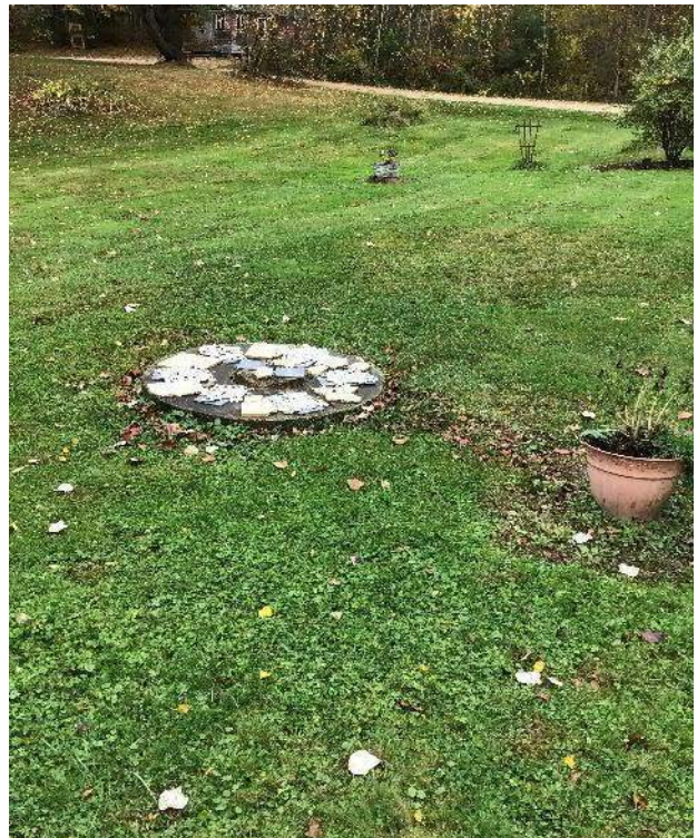
View of the location of the buried septic tank denoted by a concrete circular cover, facing South.
