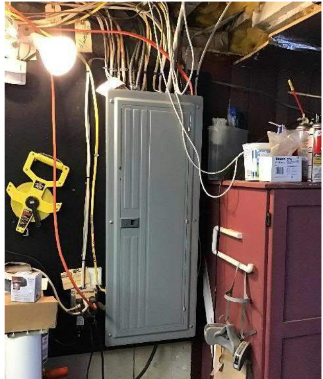
View of breaker box and surrounding wall space located on the ground floor facing Northwest.
