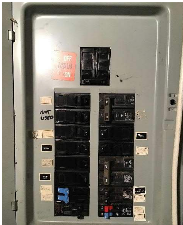
View of breaker box #1 circuit breakers and schedule adjacent to the breakers.
