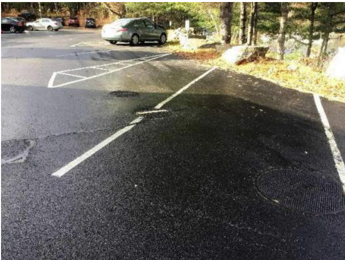
View of the location of the septic tank and manholes in the North parking lot facing West.
