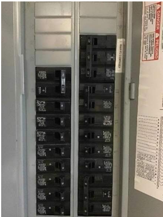
View of breaker box #1 circuit breakers.
