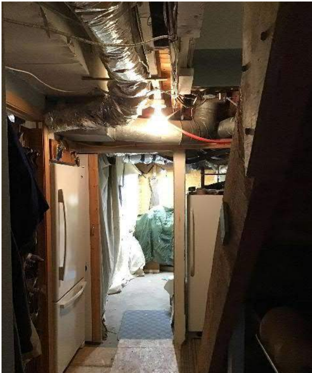
View of a hallway on the ground level leading to the room with the existing sewer lateral.
