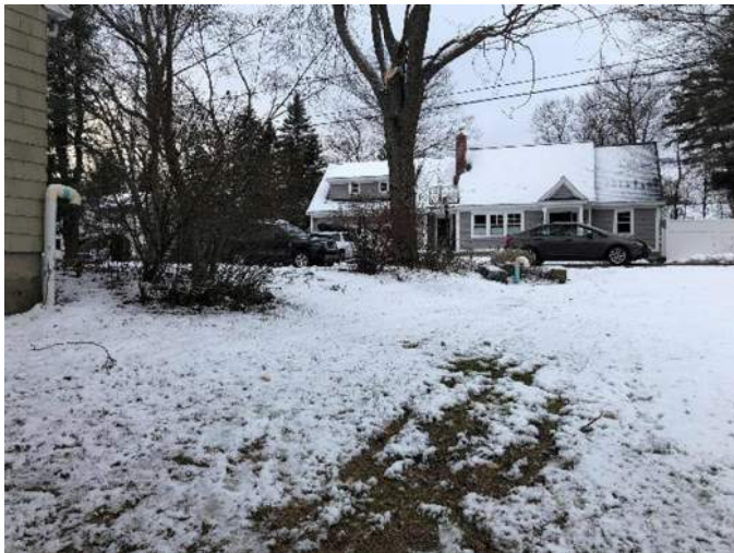
View of septic leach field in the Northwest lawn near Cliff Road facing Southwest.
