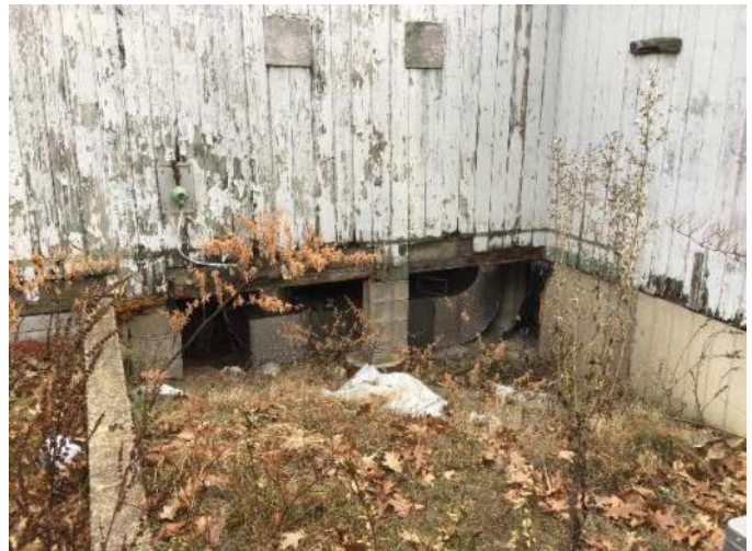
View of HVAC ducts beneath the building facing Southwest.
