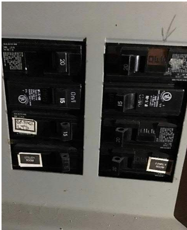
View of breaker box #2 circuit breakers with some schedule labels on the breaker switches.
