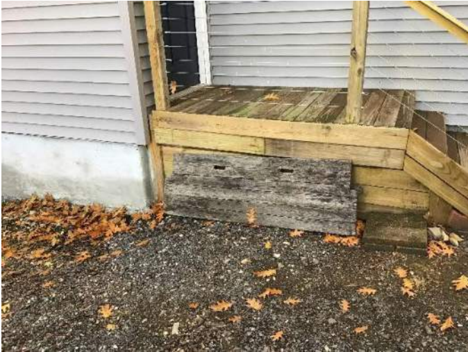
View of the wooden deck where proposed sewer service and plumbing redirecting the existing sewer lateral will be laid facing Southeast.
