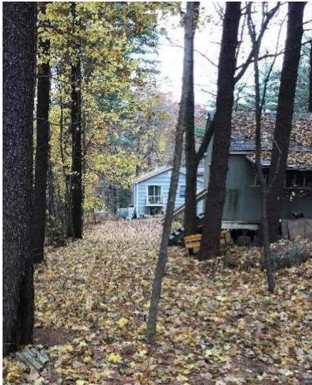
View from the leach field towards the pump station and septic tank near the house, facing Northeast.
