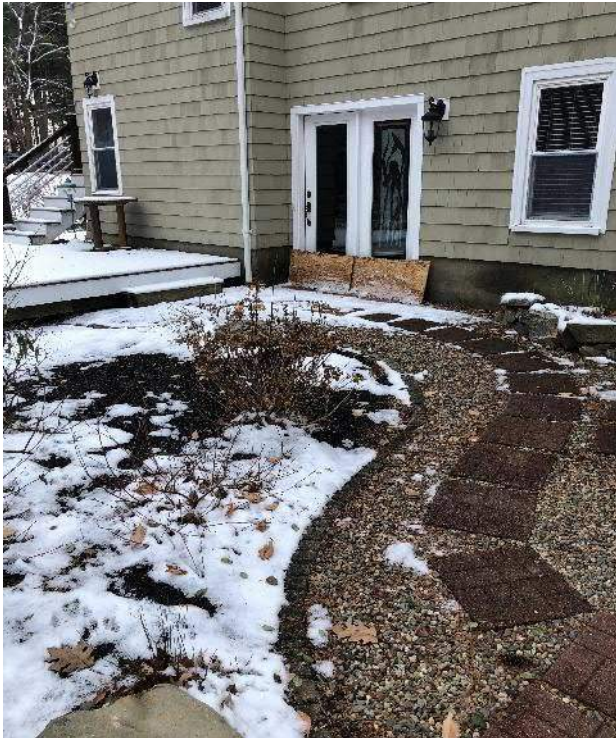
View of gravel path in the rear of the house and approximate location of the sewer lateral facing South.
