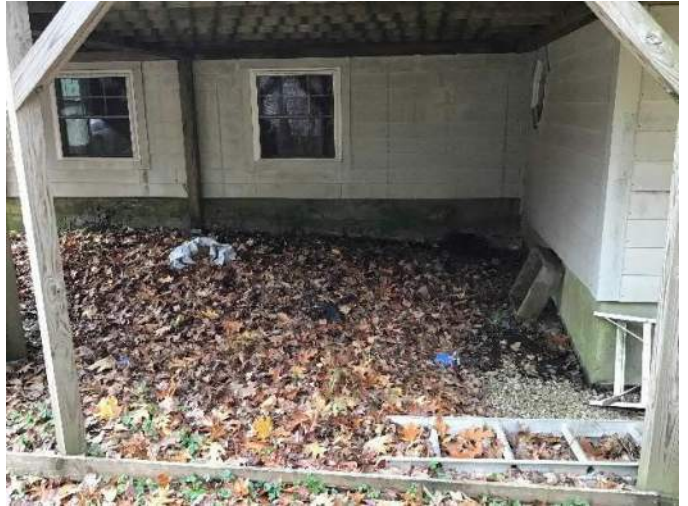
View beneath the raised wooden porch and approximate location of the buried sewer lateral facing Southwest.
