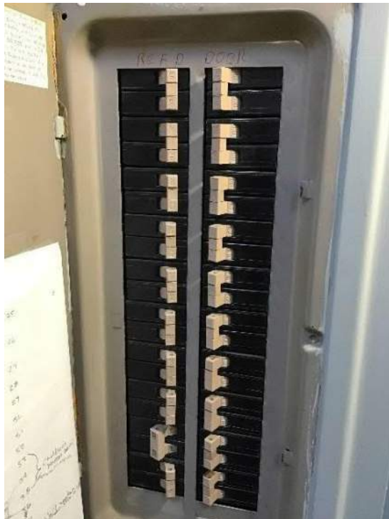
View of breaker box #2 circuit breakers located on the wall in the main lobby on the first floor.
