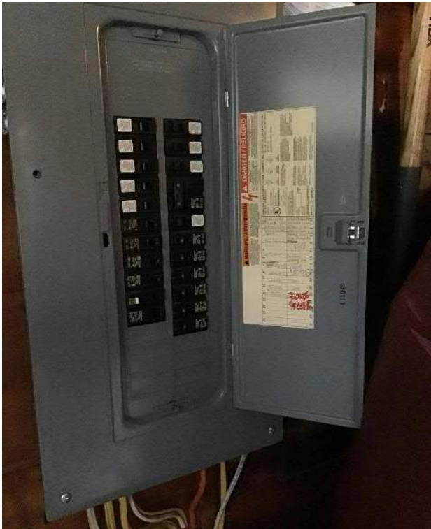
View of the breaker box located on the Southeast interior garage wall facing South.
