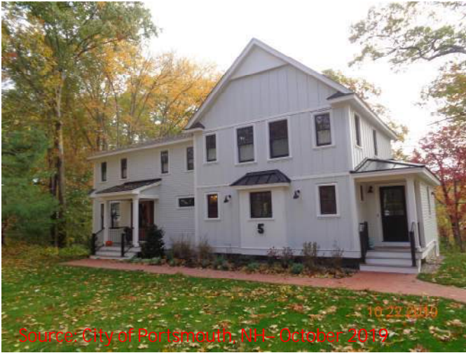
View of 5 Sagamore Grove from the front yard, facing East.
