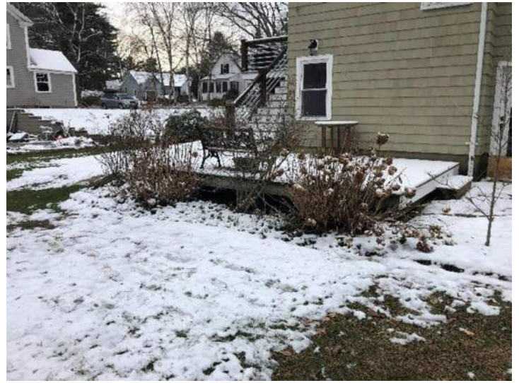
View of wooden deck on the Southeast corner of the house, facing South.
