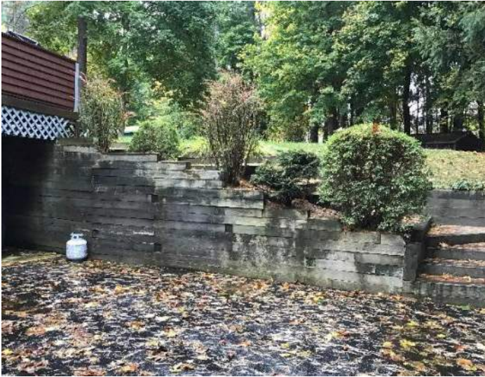
View of wooden retaining wall separating the backyard and asphalt driveway, adjacent to the garage facing Southwest.
