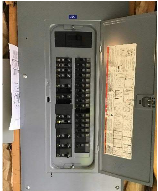
View of the breaker box with front panel cover open, facing Northwest.
