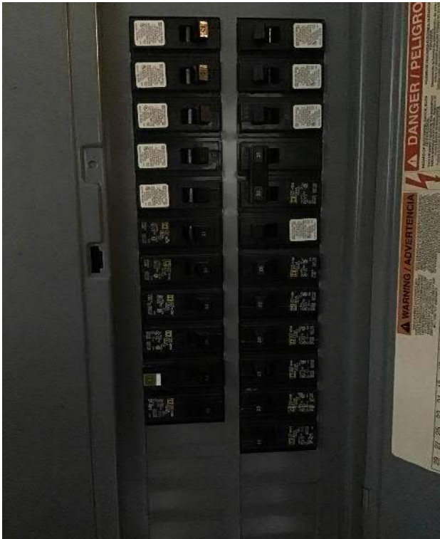
View of breaker box circuit breakers.
