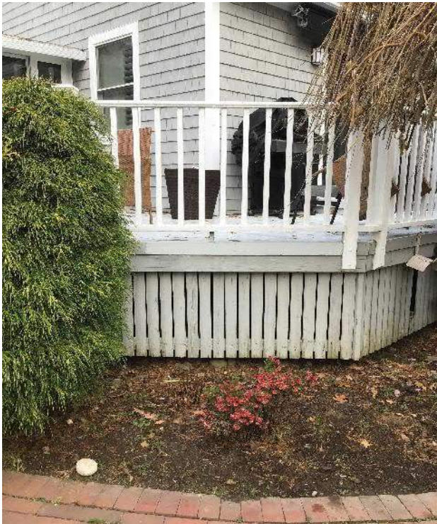
View of raised wooden deck and approximate location of the sewer lateral and septic tank underneath facing North.
