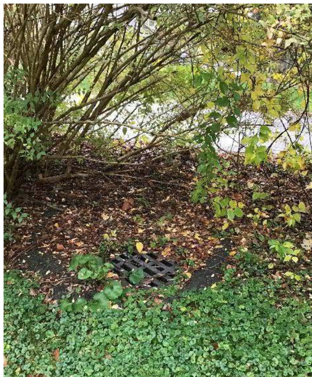
View of catch basin within the shrubs adjacent to the proposed sewer service path facing Southeast.
