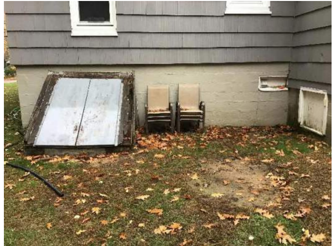
View of approximate location of buried sewer lateral and septic tank denoted by a patch of dirt facing Northeast.
