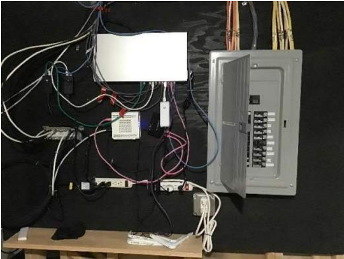
View of breaker box #2 located on a basement wall, facing North.
