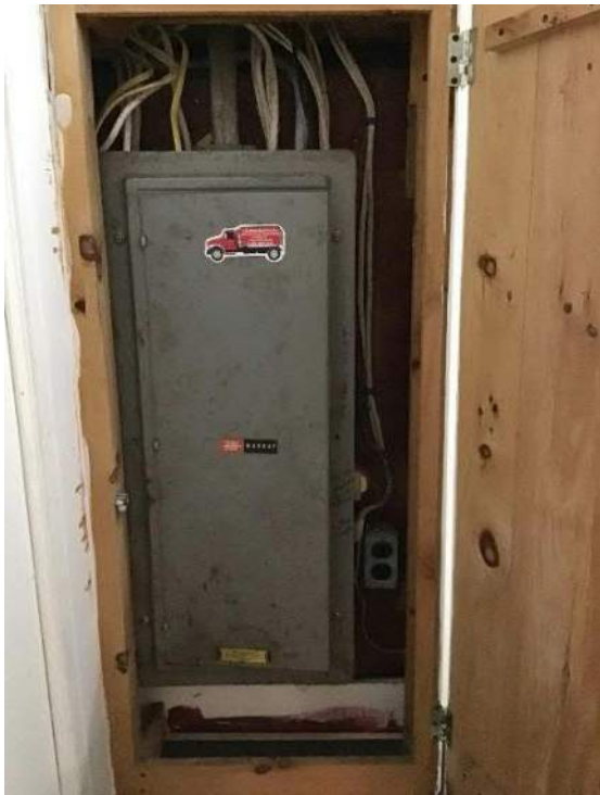
View of breaker box circuit breakers.
