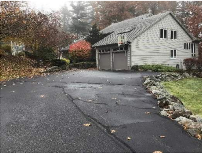
View of 272 Walker Bungalow Road from the end of the driveway facing Southeast.
