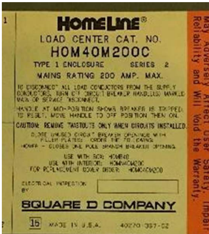
View of breaker box #2 model information and specifications.
