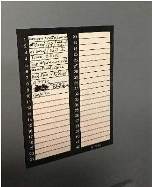
View of breaker box #5 schedule.
