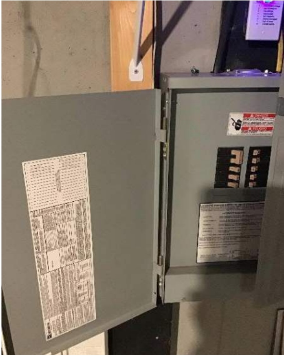
View of transfer switch with panel cover open.
