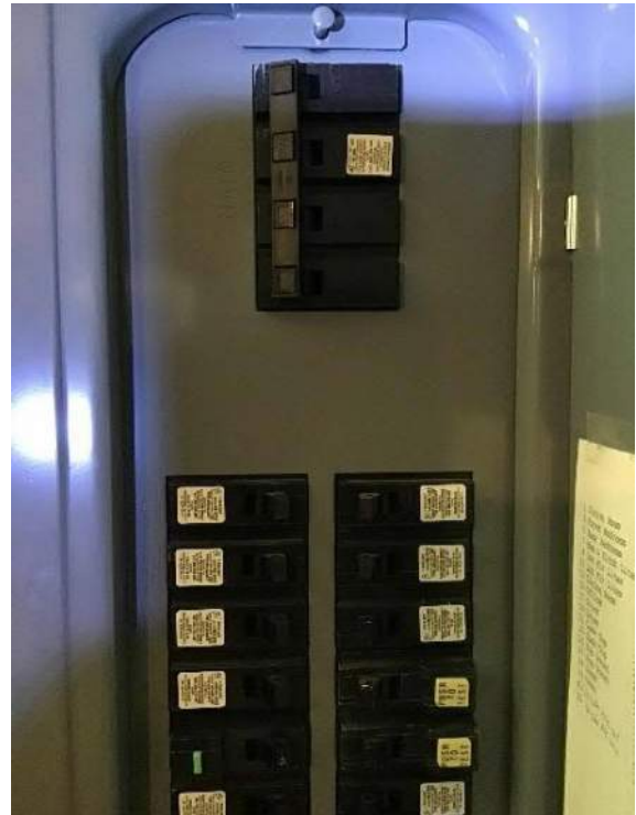
View of breaker box #2 circuit breakers.
