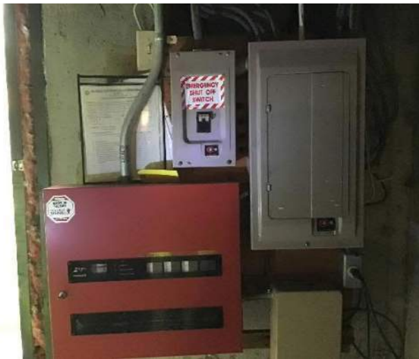
View of the breaker box and fire suppression system located to the right of the basement steps facing West.
