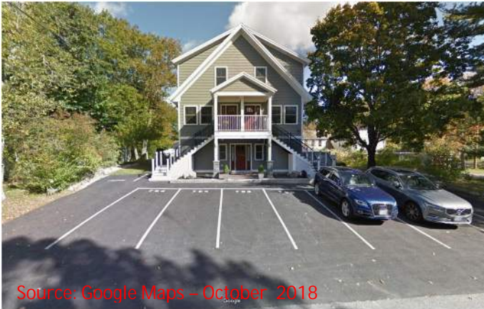
View of 792, 794, 796 Sagamore Avenue and asphalt parking lot from the road facing Northwest.
