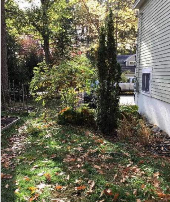
View of buried septic tank and lateral at the bottom of the frame standing adjacent to exterior garage wall facing Southwest.
