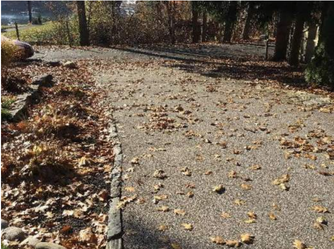
View of the asphalt driveway, granite curb and shrubs, facing South.
