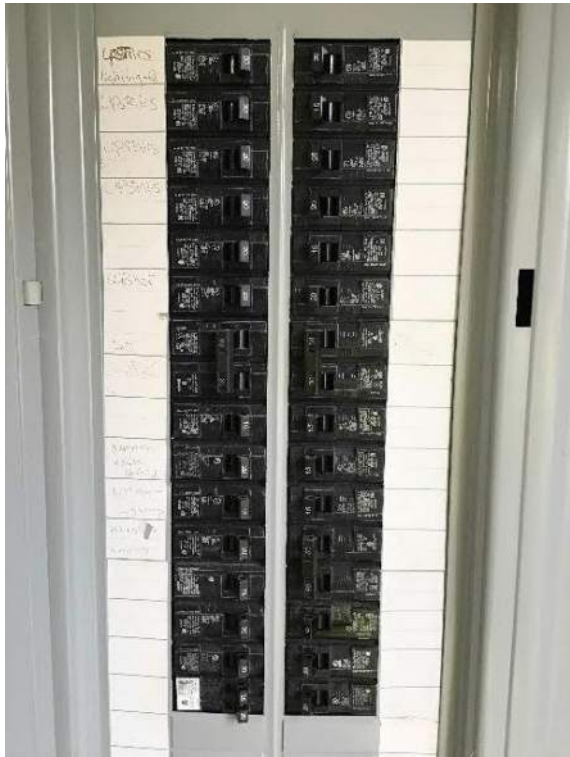
View of Siemens breaker box circuit breakers and schedule adjacent to breaker switches facing
