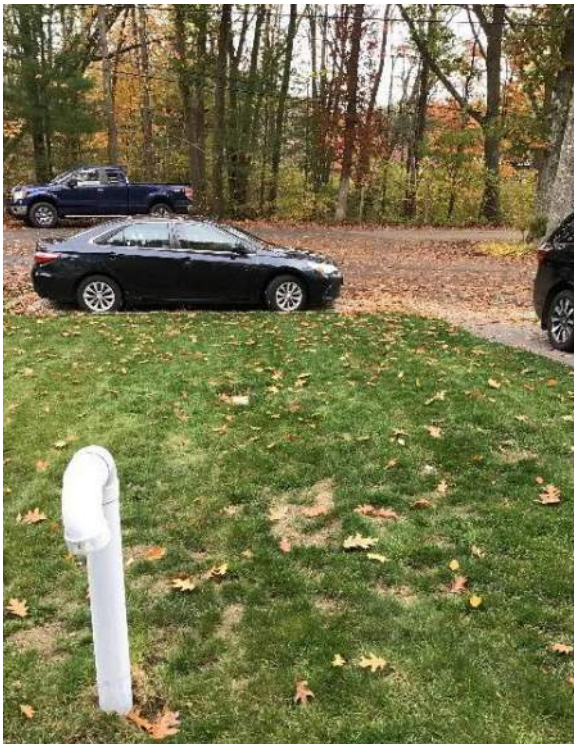
View of proposed sewer service pathway towards the road through a gravel driveway facing South.
