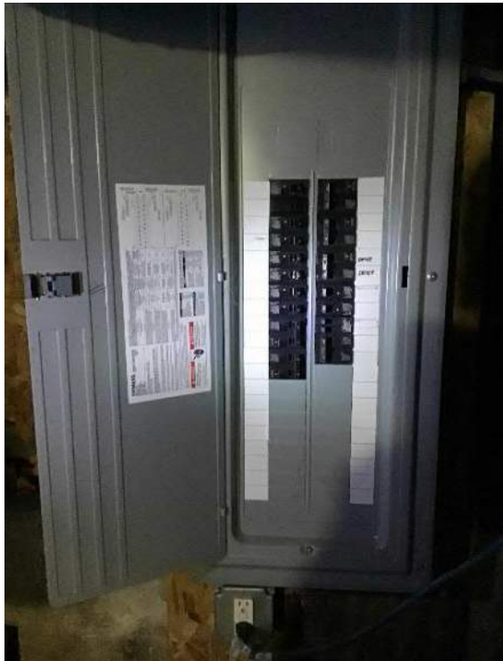
View of breaker box #1 located in the basement facing Southwest.
