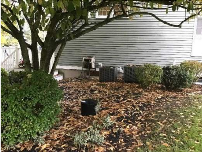
View of air conditioning units and propane tank on the East side of the house near proposed excavation, facing West.
