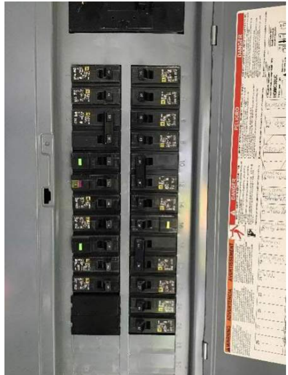
View of the breaker box open and circuit breakers facing Northwest.
