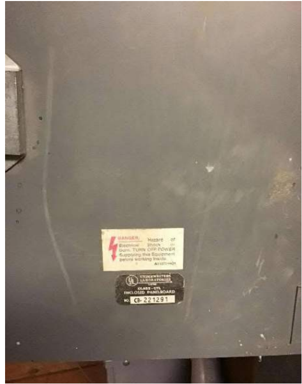
View inside of breaker box #1 panel cover with model number.
