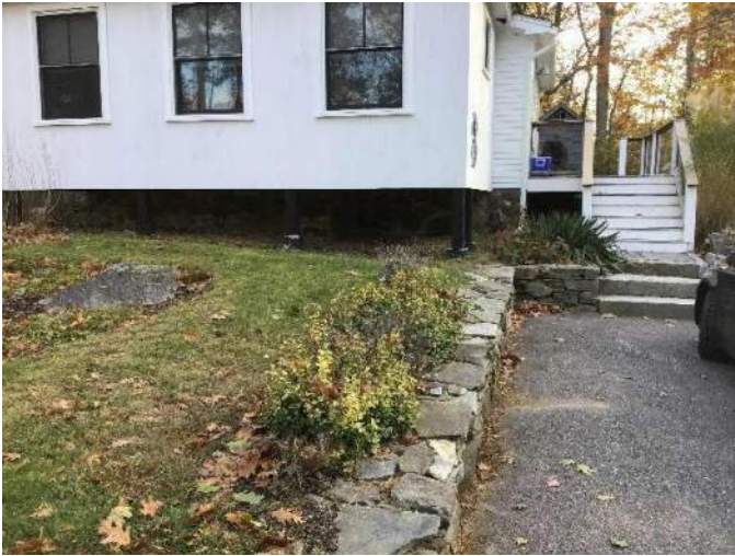
View of 3 Sagamore Grove and retaining wall around the asphalt driveway facing South.
