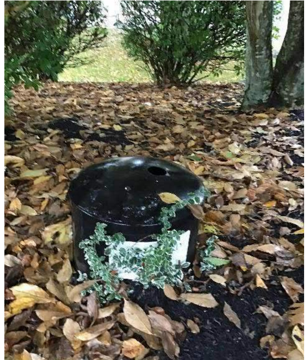
View of propane tank cover within the garden, facing Southwest.
