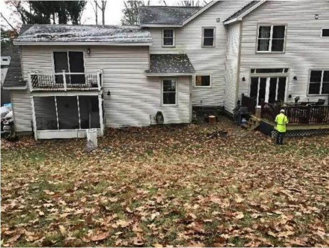
View of the rear side of the house and backyard from the top of the hill facing South.
