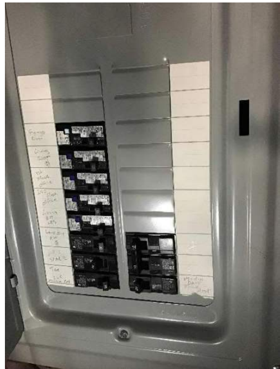
View of breaker box #2 (Siemens) circuit breakers and schedule, located near breaker box
