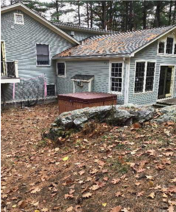
View of exposed ledge near approximate septic tank location, facing East.
