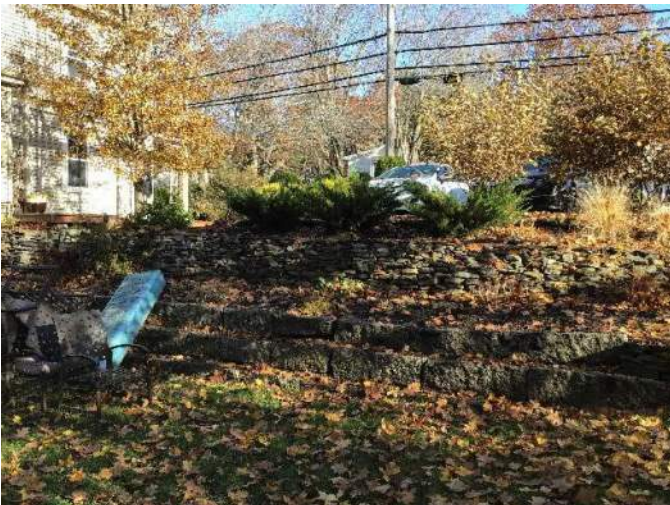
View of retaining wall from the back yard sloping up to the asphalt driveway facing North.
