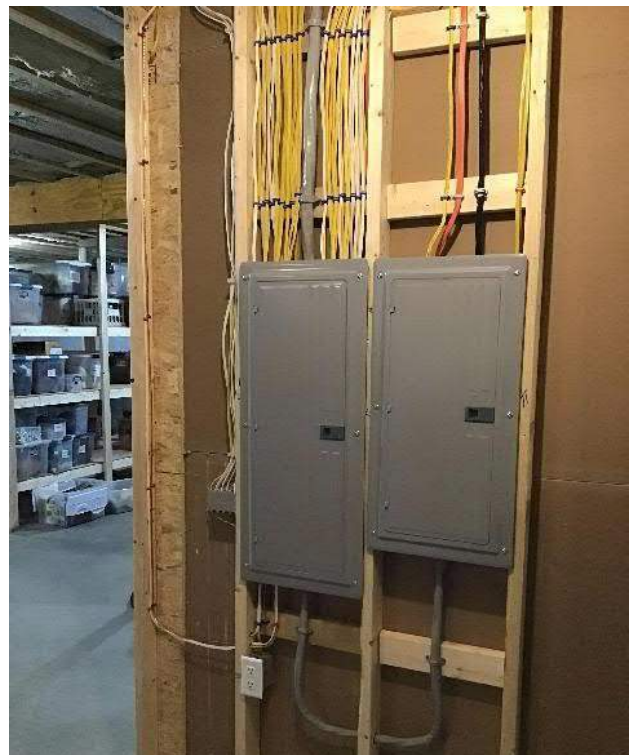
View of two breaker boxes (#1 is left) and surrounding wall space facing West.
