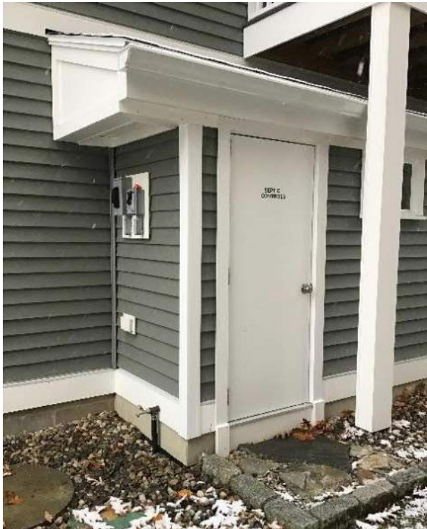
View of two control panels on the side of a room with a door marked "Septic Controls" facing South.
