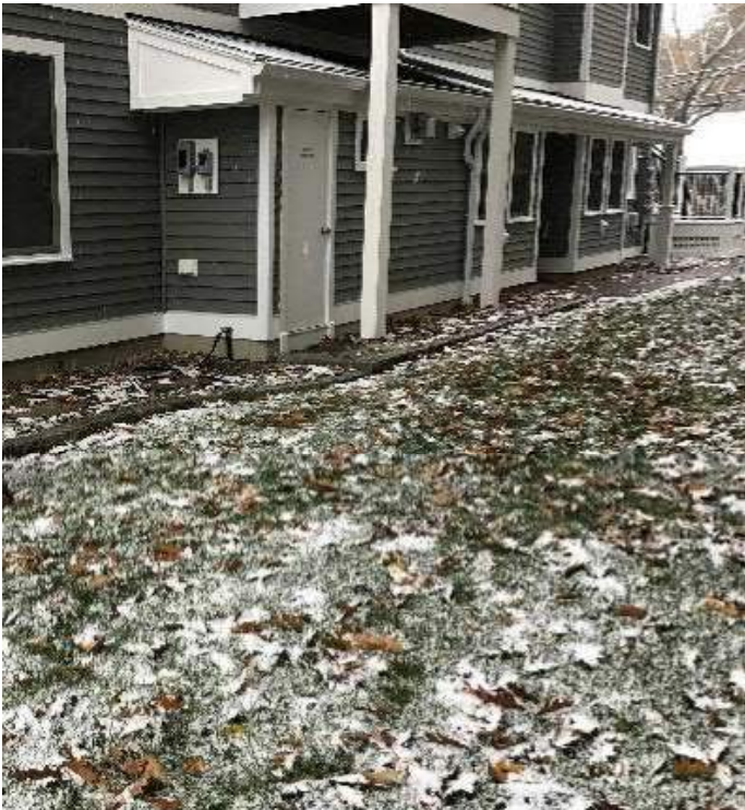
View of stone edging along the Northwest side of the building, facing South.
