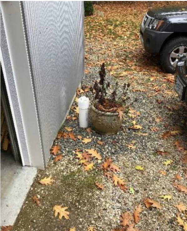
View of buried sewer lateral running under the garage floor to the septic tank in the driveway, facing West.
