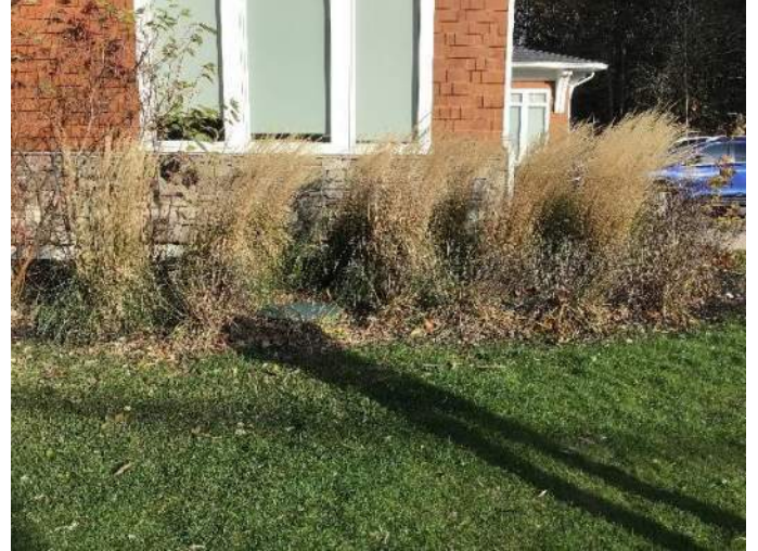
View of West exterior wall and shrubs and landscaping facing East.
