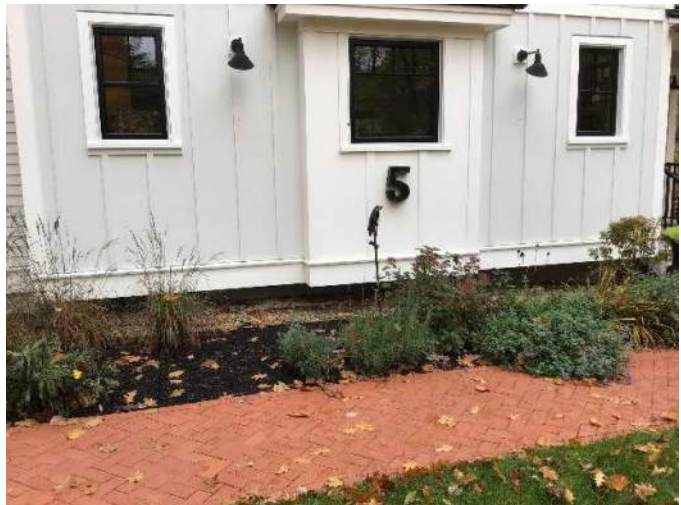
View of approximate location of buried sewer lateral underneath the stone, shrubs, and brick, facing Southeast.
