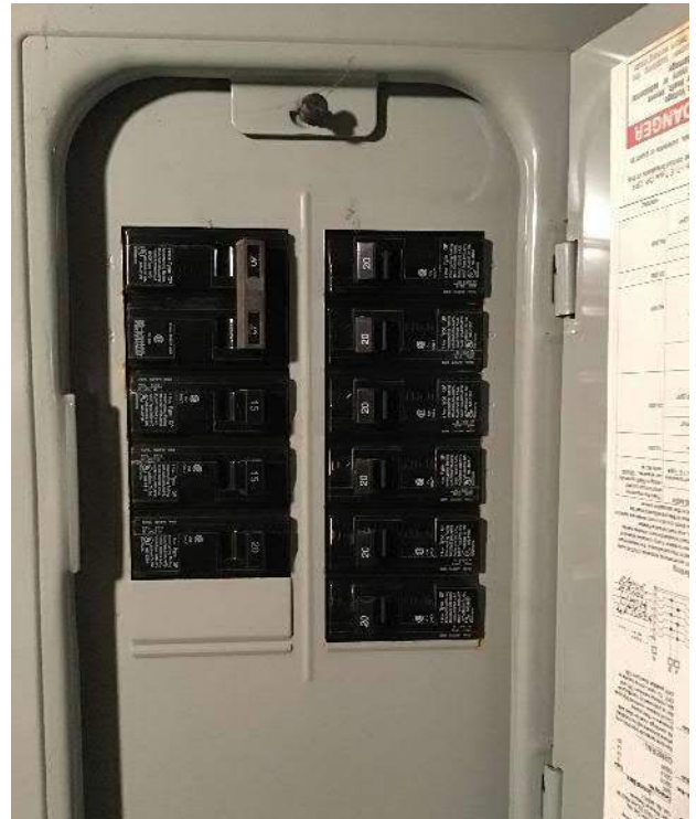
View of breaker box #2 (Siemens) circuit breakers.
