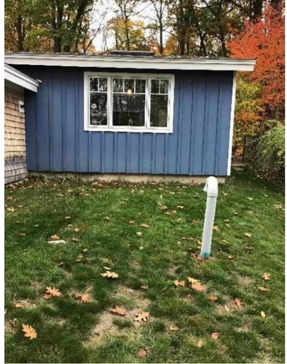
View of the location of the buried septic tank and proposed sewer service path facing North.
