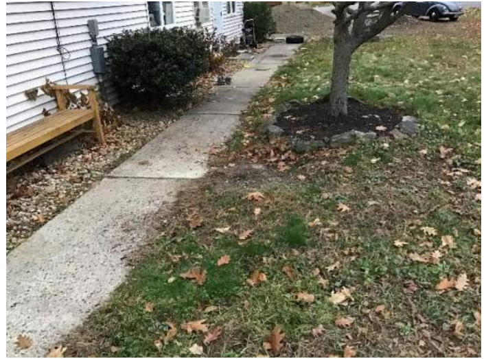
View of concrete walkway on the South side of the house facing Northeast.
