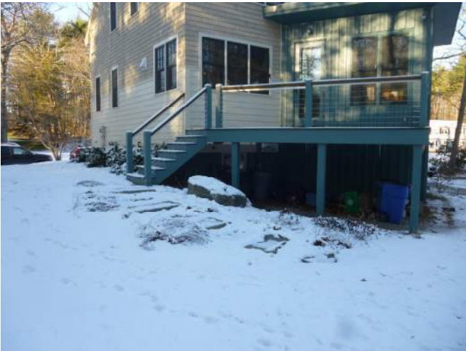
View of raised wooden porch in the rear of the house with wooden stairs near the sewer lateral, facing Southwest.
