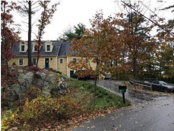
View of 11 Sagamore Grove property from Sagamore Grove facing Northeast
