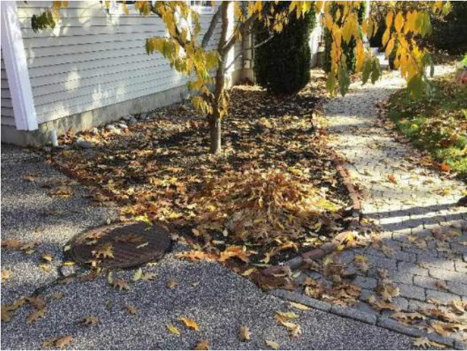
View of a manhole cover to access septic tank underneath the asphalt driveway and small tree, facing Northeast.
