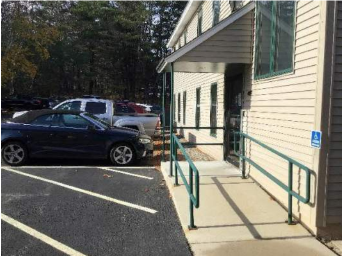
View of the Southwest exit and exterior location of breaker box #4 and #5 facing West
