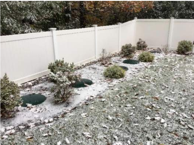
View of septic tank location and five tank caps along the fence facing North
