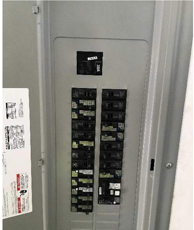
View of breaker box #1 (Siemens) circuit breakers.
