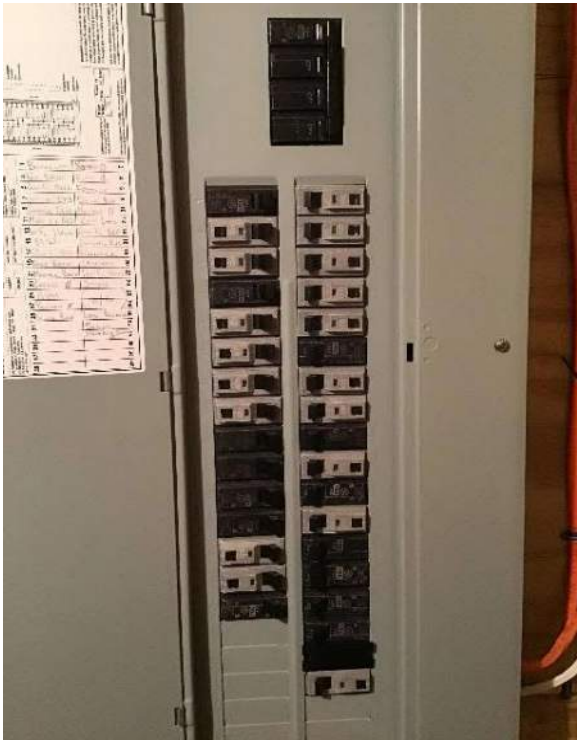
View of breaker box circuit breakers.
