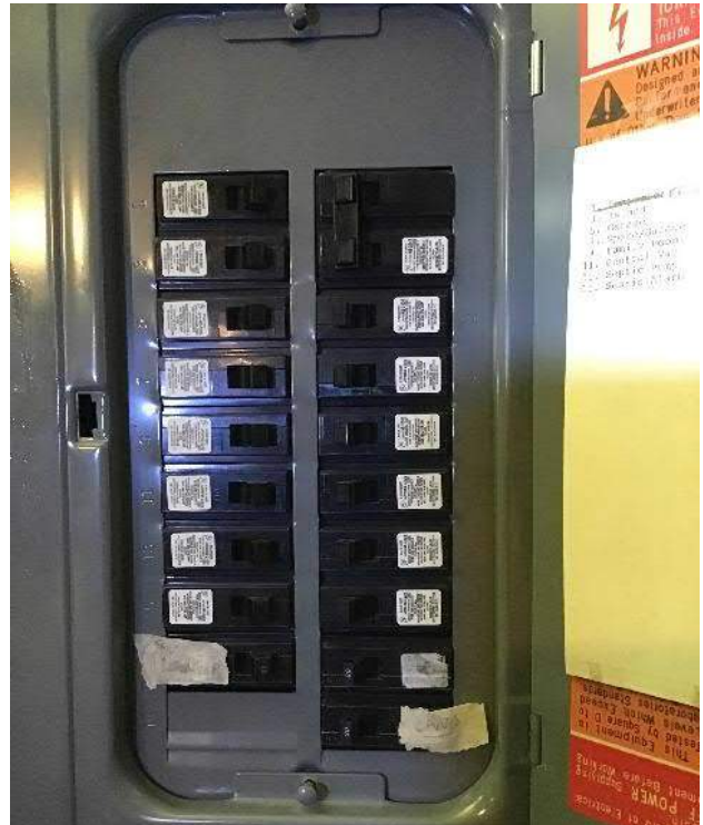
View of breaker box #1 circuit breakers.
