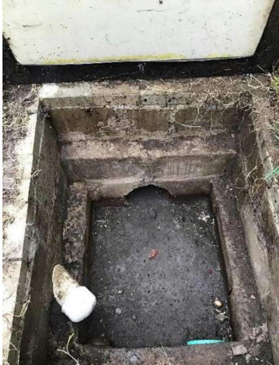
View inside drain manhole in the yard facing North.
