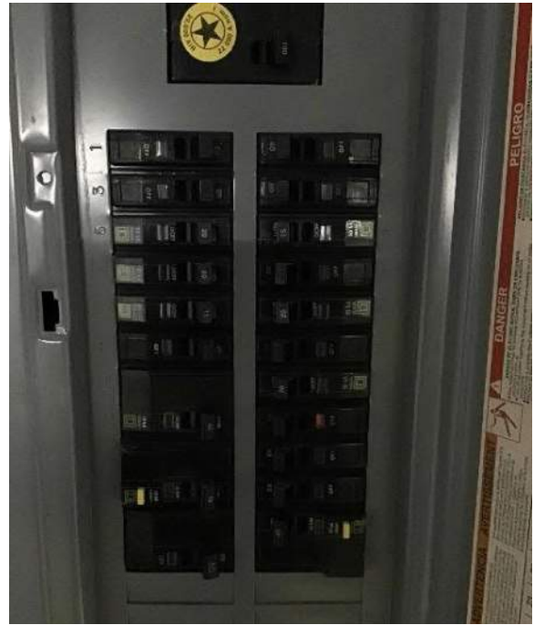
View of 100A breaker box #2 circuit breakers, located on the East foundation wall, facing East.
