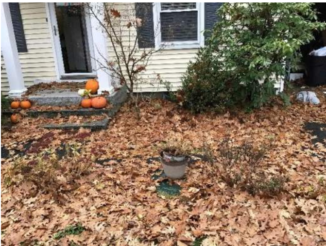
View of approximate buried sewer lateral location and pump station cap covered by a flowerpot facing Southwest.
