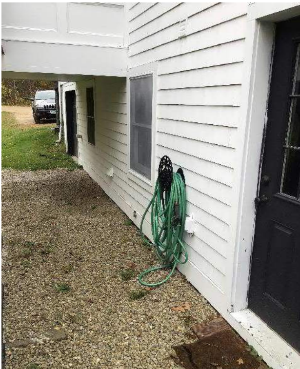
View of approximate buried sewer lateral location and pebbles spread along the house facing Southwest.
