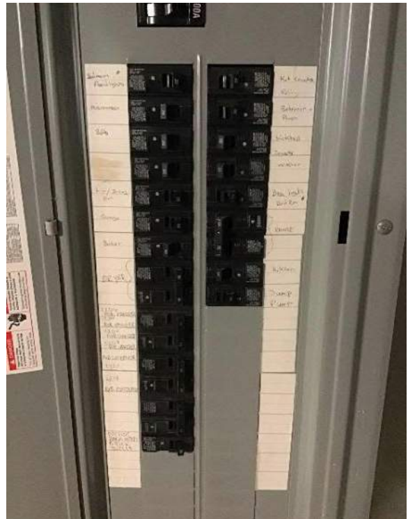
View of 200A Siemens breaker panel and schedule adjacent to breaker switches.
