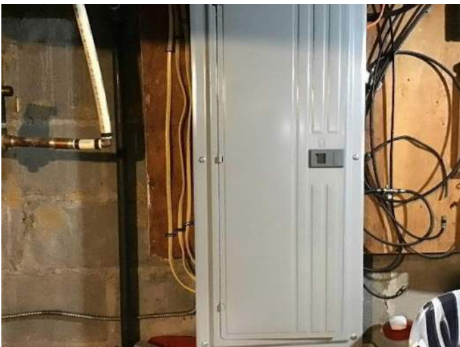
View of the breaker box and surrounding wall space located in the basement, facing Southeast.
