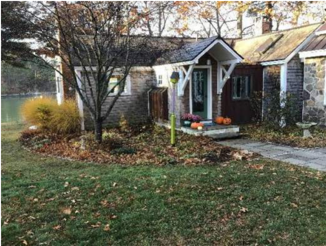
View of 238 Walker Bungalow Road from the yard facing Southwest.
