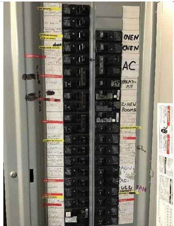
View of the circuit breakers and schedule adjacent to the breaker switches.
