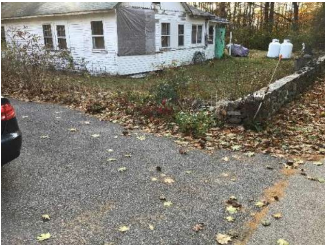
View of retaining wall crossing the proposed sewer service path facing West.
