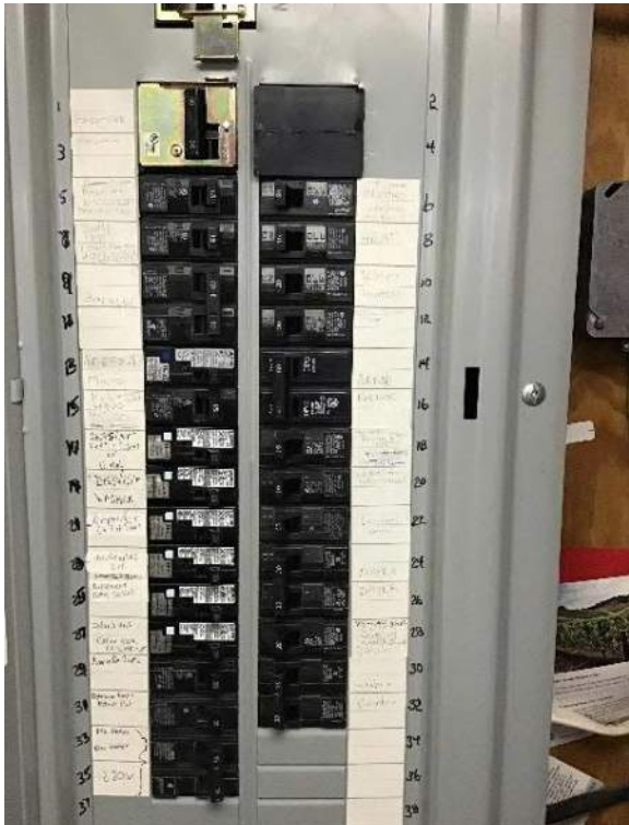
View of Siemens breaker box circuit breakers and schedule adjacent to the breaker switches.
