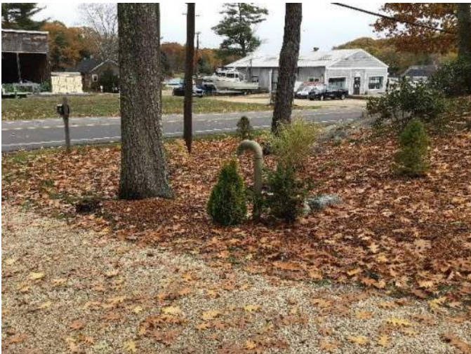
View of PVC vent pipe and shrubs on the East side of the driveway, facing Northeast.
