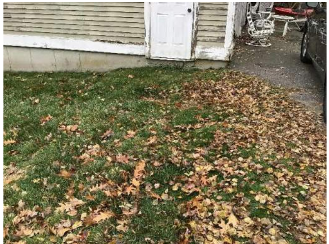
View of the approximate location of the buried sewer lateral leading from the house facing Southwest.
