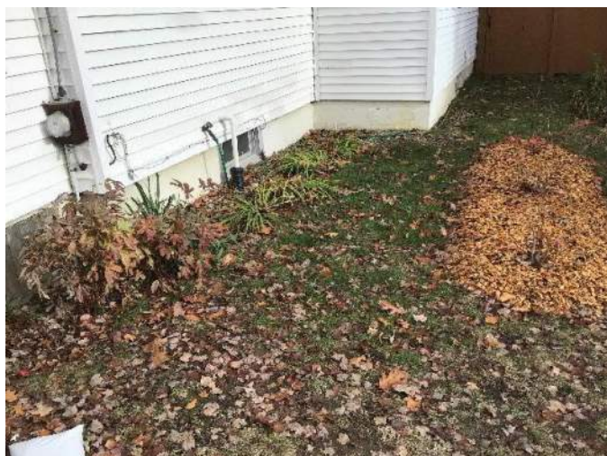
View of leach field and small shrubs along the foundation facing Northeast.
