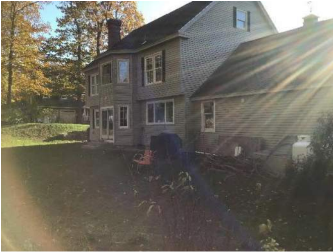
View of the back of the house and backyard facing South.
