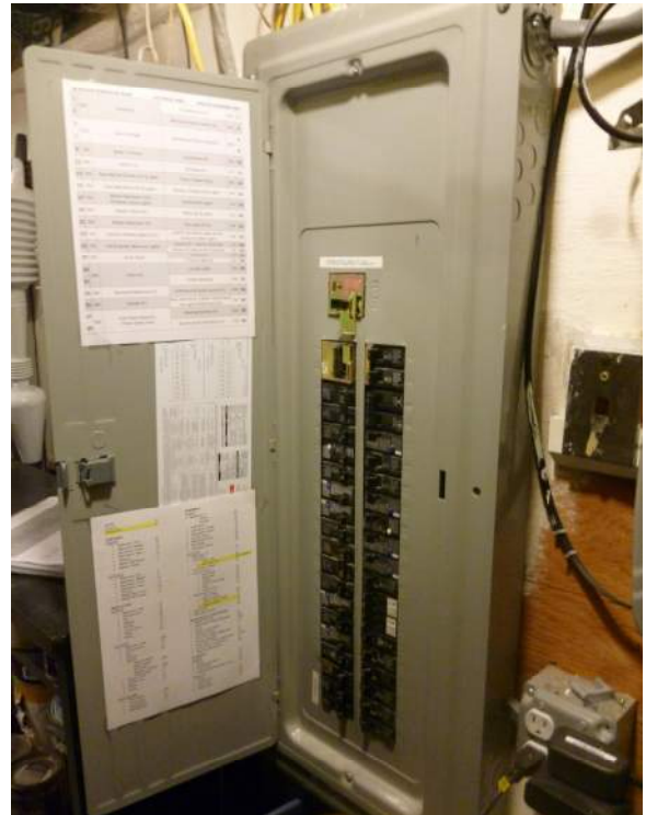
View of breaker box front panel and circuit breakers facing North.
