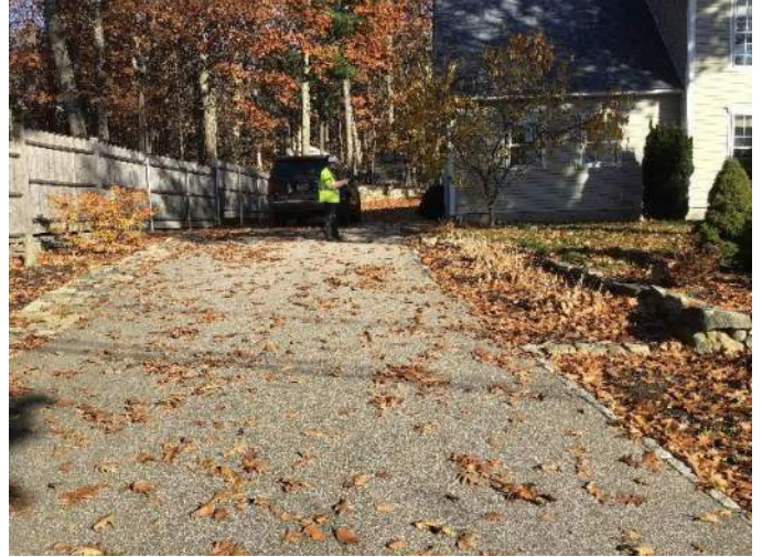
View of the asphalt driveway and proposed sewer service path facing North.
