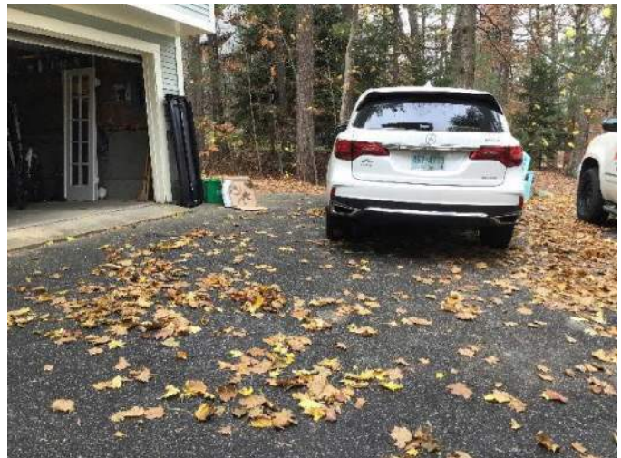
View of asphalt driveway and proposed sewer service path through the driveway, facing Northwest.
