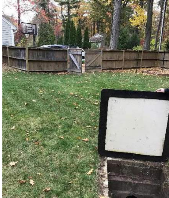
View of buried storm drain pipe running under the fence and access hatch facing North.
