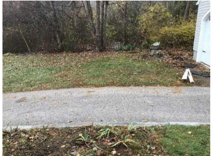
View of asphalt driveway and granite curb along the edge adjacent to the front lawn facing Southwest.
