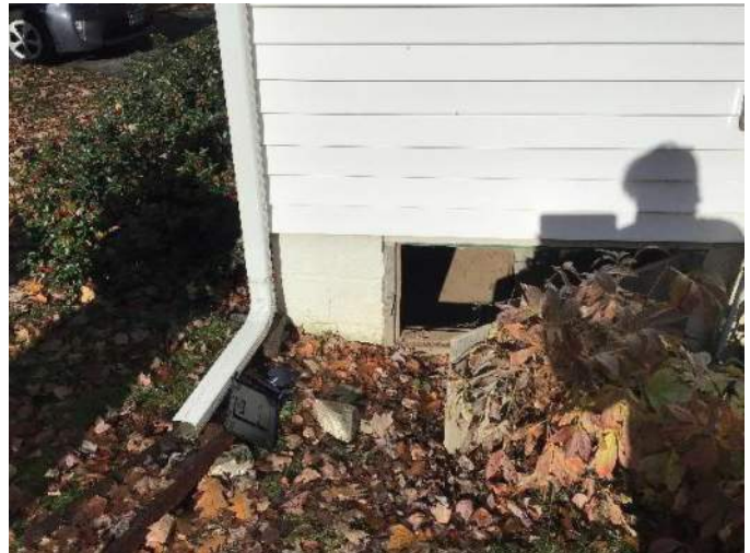
View of gutter splash block and crawlspace access under the front porch, facing Northwest.
