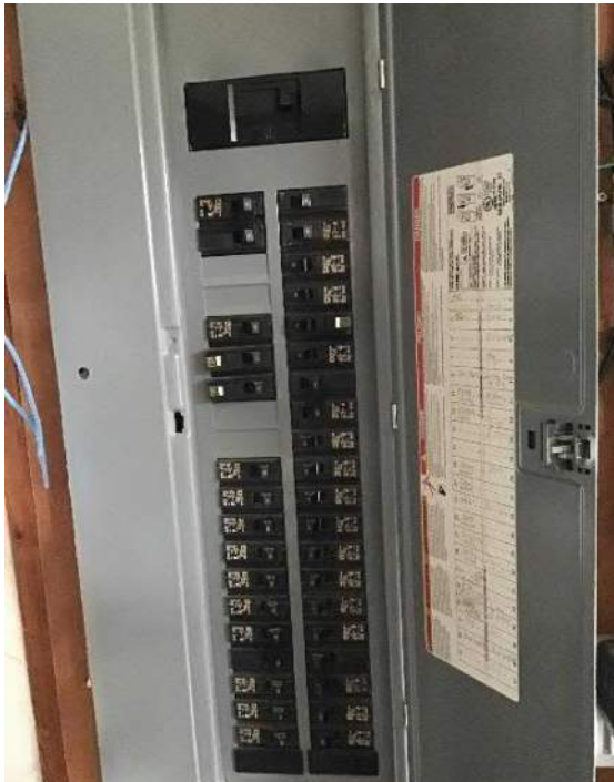
View of Homeline breaker box front panel and circuit breakers.
