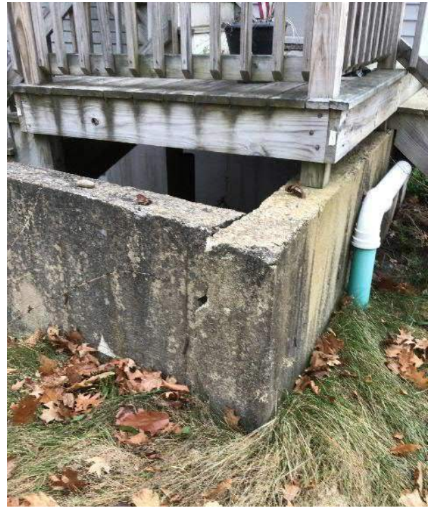
View of second crack in the concrete retaining wall due to overturning facing Southwest.
