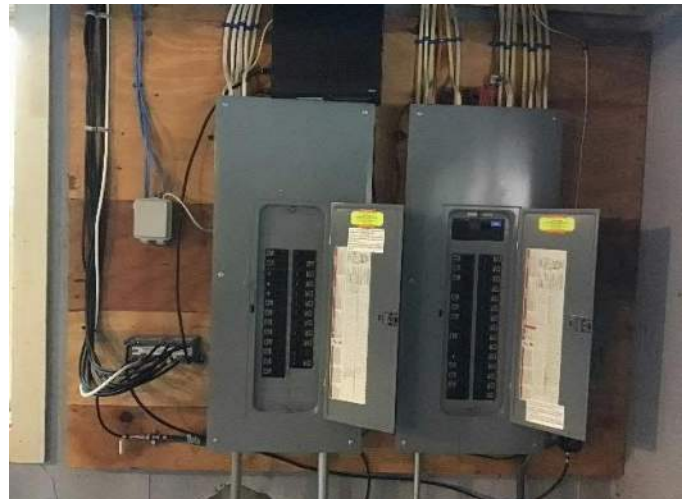
View of breaker boxes (#1 on left) and surrounding wall space located in the garage, facing Northeast.
