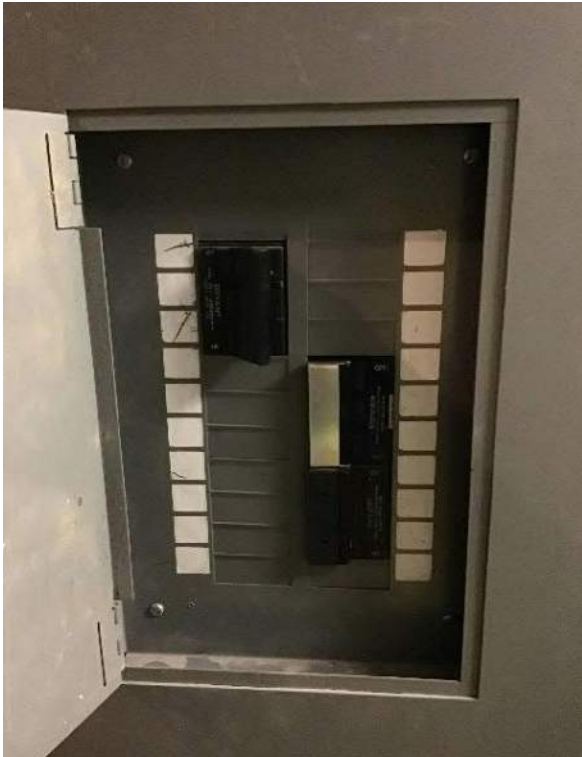
View of breaker box #1 panel and circuit breakers.
