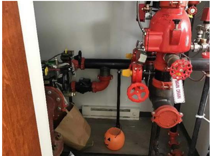
View of fire suppression system in a closet on the West section of the building facing North.
