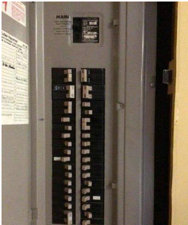
View of breaker box #3 circuit breakers.
