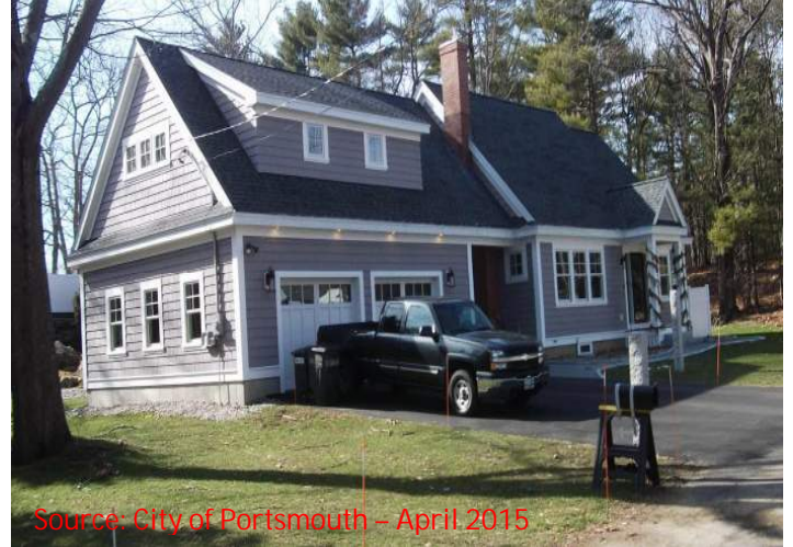
View of 96 Cliff Road from the street facing Northwest.
