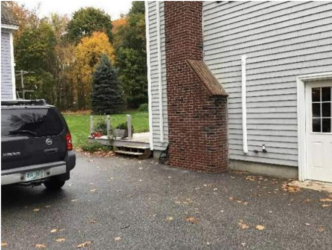
View of approximate location of buried sewer lateral adjacent to the masonry chimney, facing Northwest.
