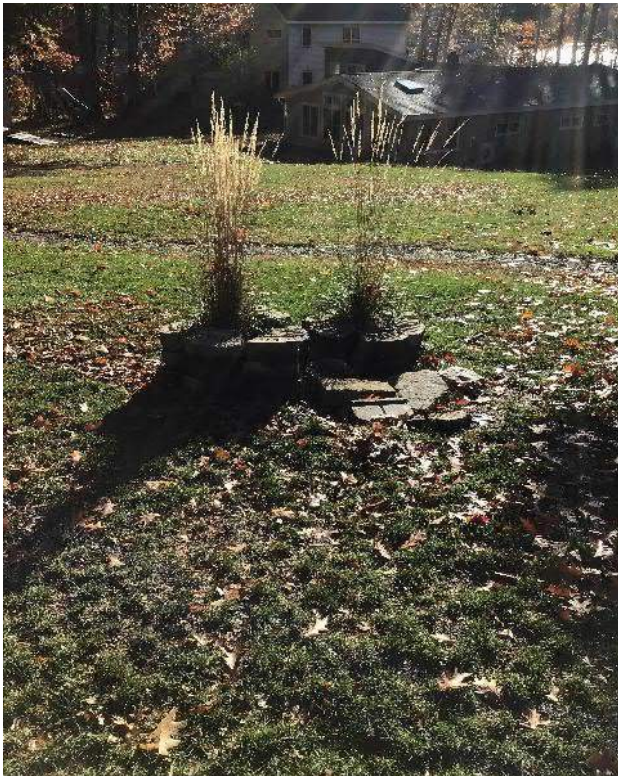
View of the location of the buried septic tank in the backyard facing Southeast.
