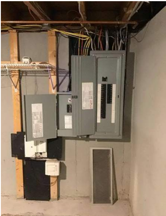
View of breaker box, transfer switch and their surrounding wall space facing Southeast.
