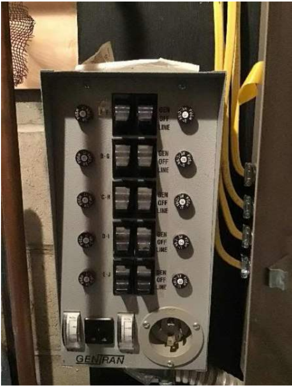
View of manual transfer switch front panel to the left of the breaker box.
