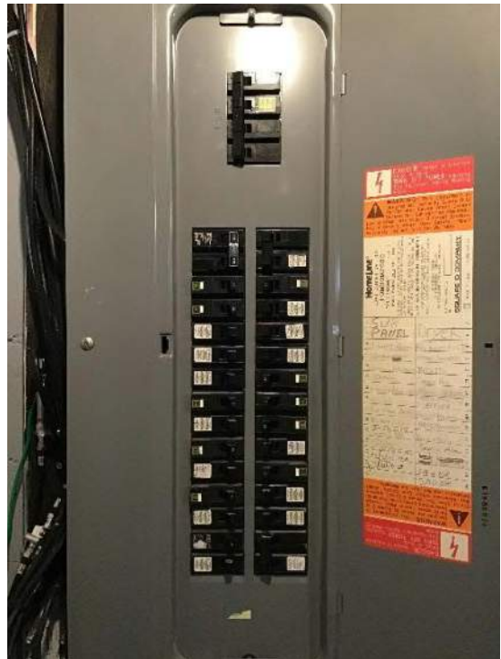
View of breaker box #1 circuit breakers facing Northwest.
