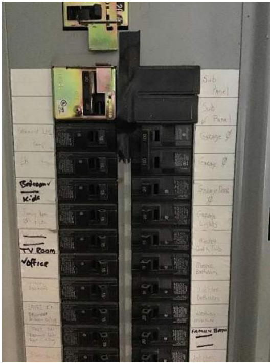
View of 200A breaker box #1 (Siemens) breakers and schedule adjacent to breaker switches.
