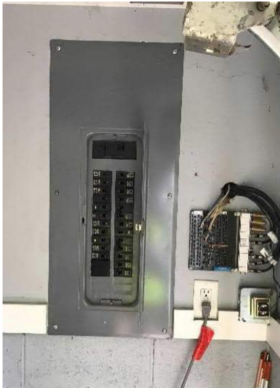
View of the breaker box and wall space adjacent to the garage door facing Southeast.
