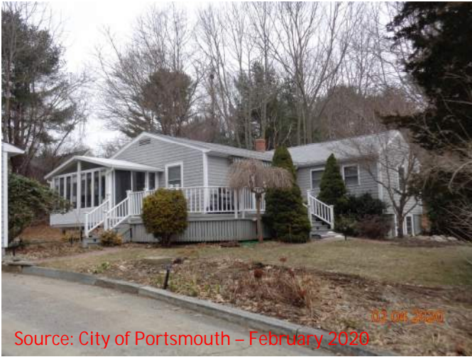
View of 911 Sagamore Avenue from the end of the driveway, facing North.
