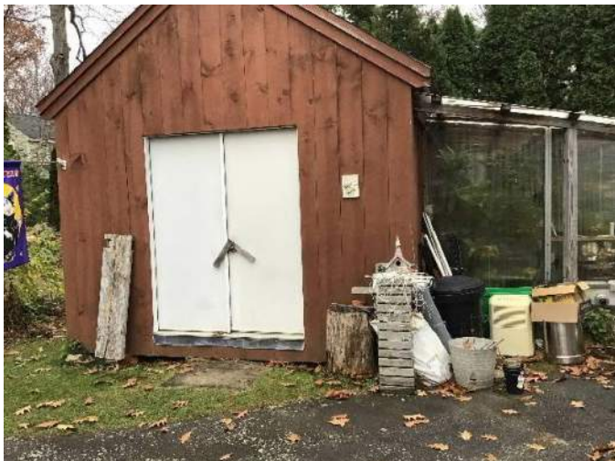
View of storage shed next to the driveway; water service runs beneath the shed to the house, facing Southeast.
