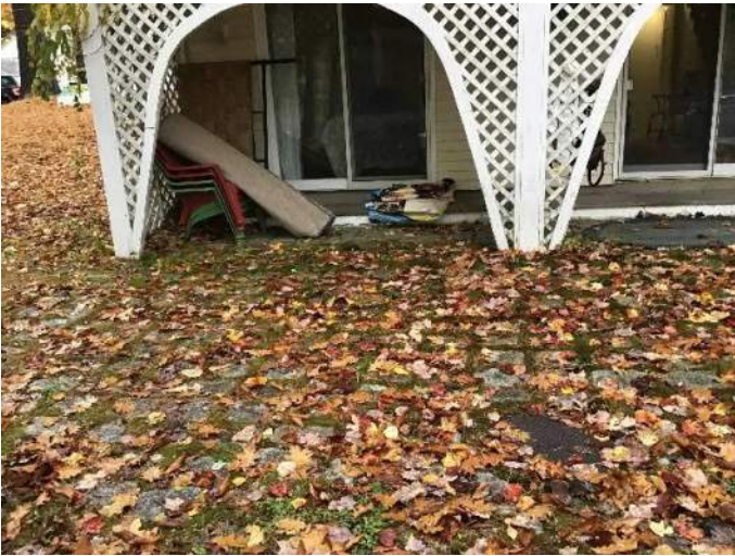
View of cobblestone patio and location of the buried septic tank facing South.
