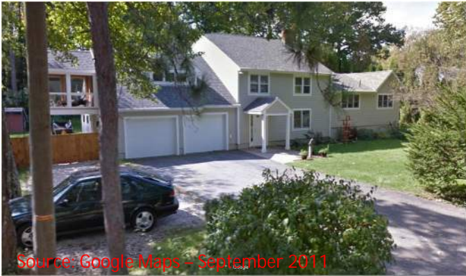
View of 140 Walker Bungalow Road from Walker Bungalow Road facing West.
