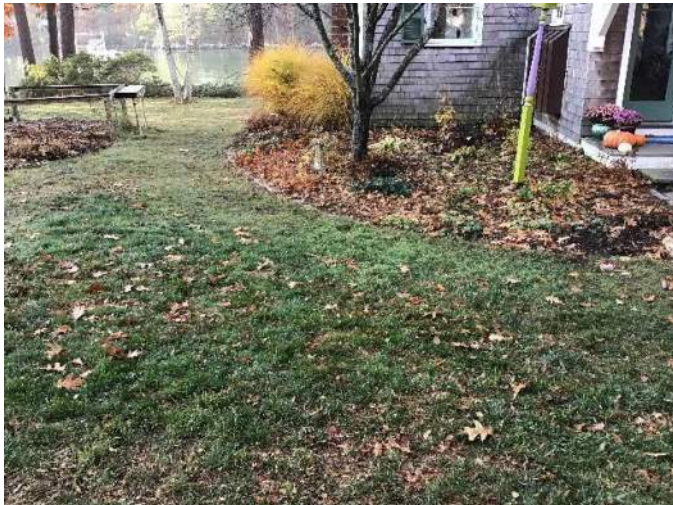
View of tree and landscaping on top of approximate sewer lateral location facing Southwest.
