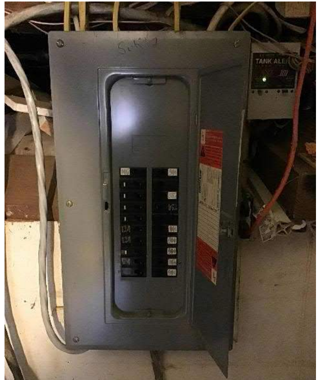
View of breaker box #1 in unfinished basement adjacent to PVC sewer lateral facing Northeast.
