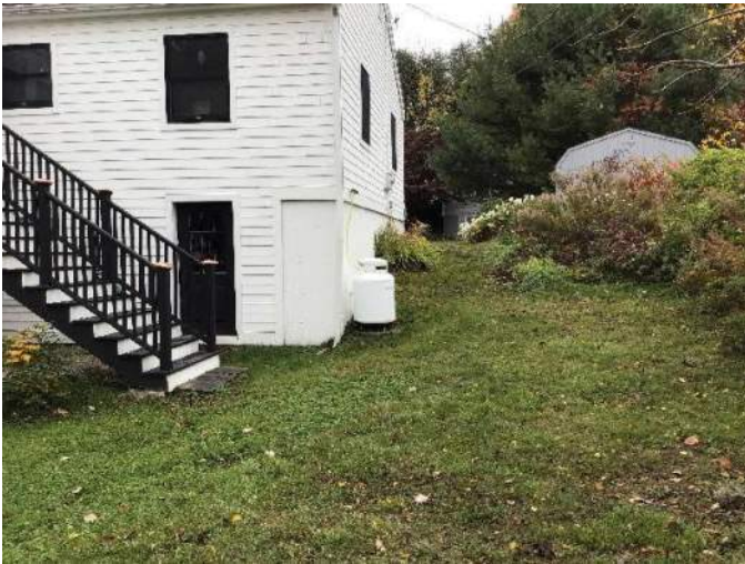
View of the Northeast side of the house and basement door facing Northwest.
