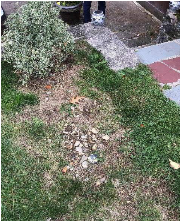
View of approximate location of cap for septic tank adjacent to a concrete retaining wall facing Northeast.
