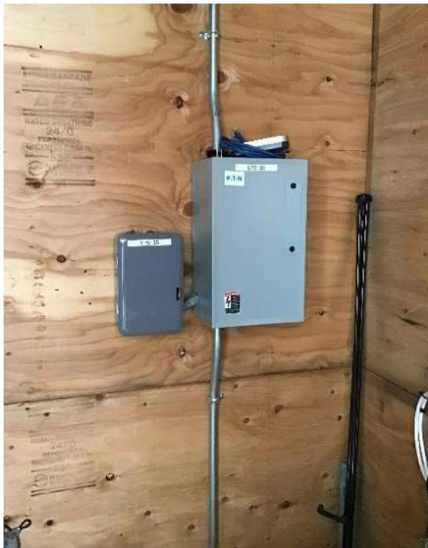
View of breaker box #3 labeled LP2-35 and LP2-36 left to right located in the same closed as boxes #1 and #2 facing North.
