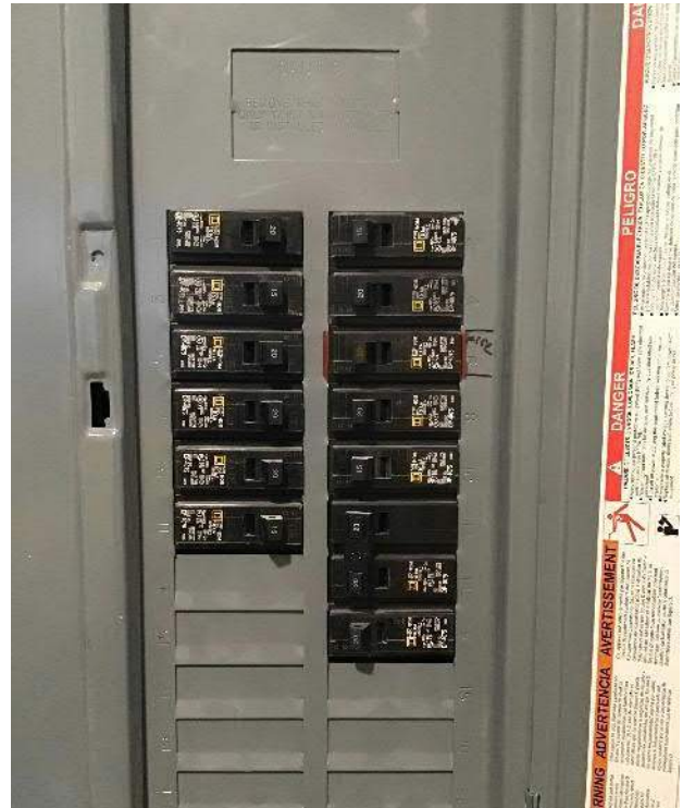
View of breaker box circuit breakers.
