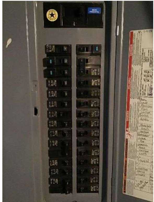
View of breaker box #1 circuit breakers.
