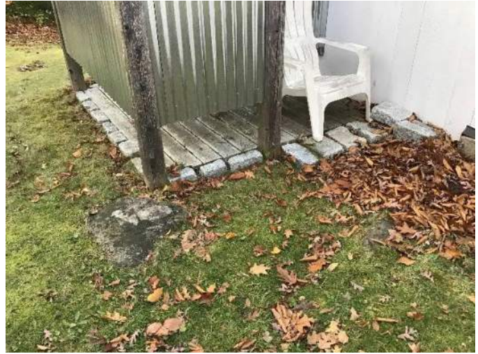
View of exposed ledge in the backyard next to the outdoor shower, facing Northeast.
