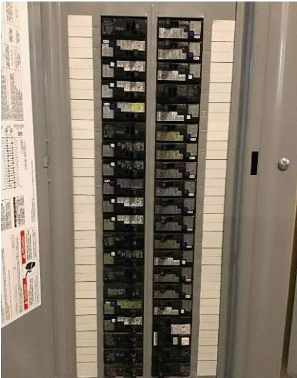
View of breaker box #1 circuit breakers.
