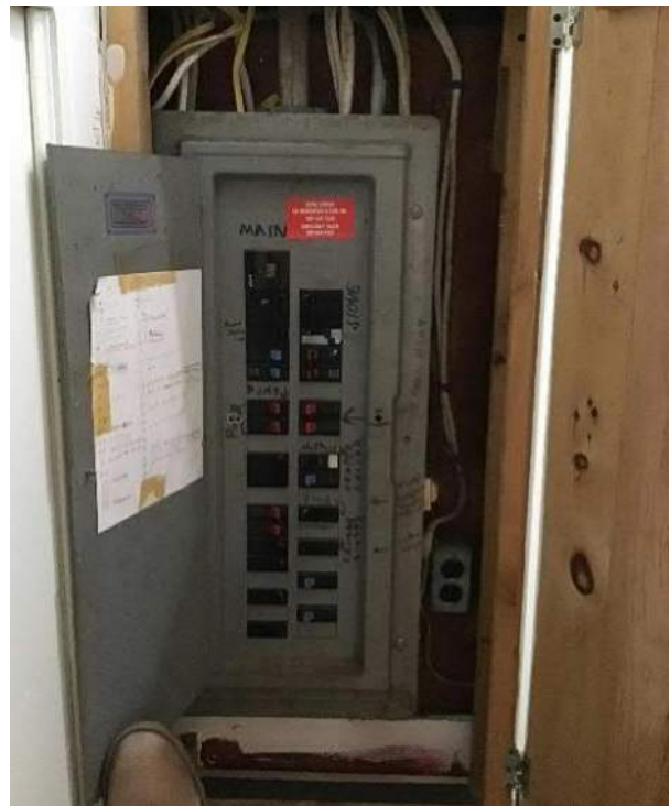
View of breaker box circuit breaker schedule on the inside of the panel cover.
