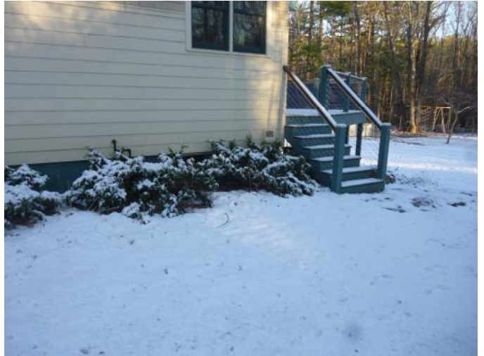
View of the East corner of the house and approximate sewer lateral location covered by shrubs facing North.
