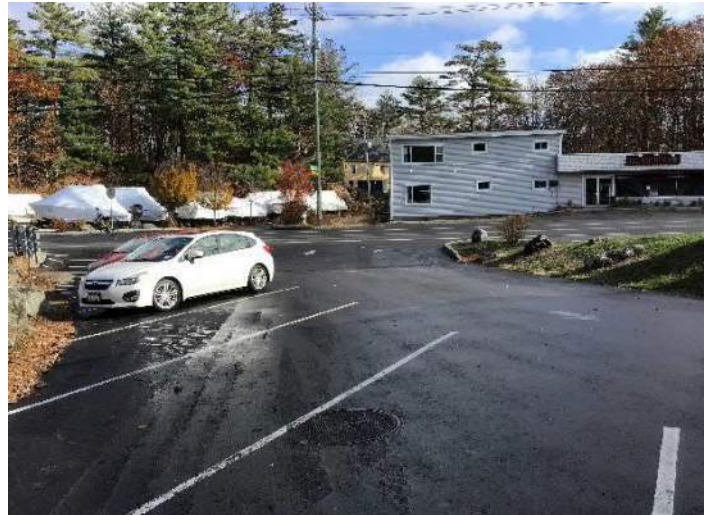
View of the proposed sewer service path through the asphalt parking lot towards Sagamore Avenue facing East.
