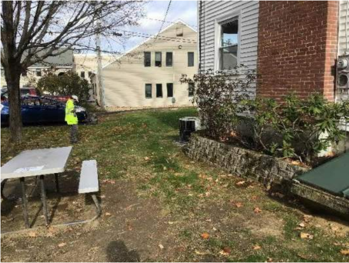
View of the West yard looking towards the Northwest corner of the building and septic tank in the North yard facing North.
