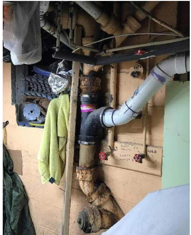
View of exposed cast iron sewer lateral and surrounding plumbing, facing North.
