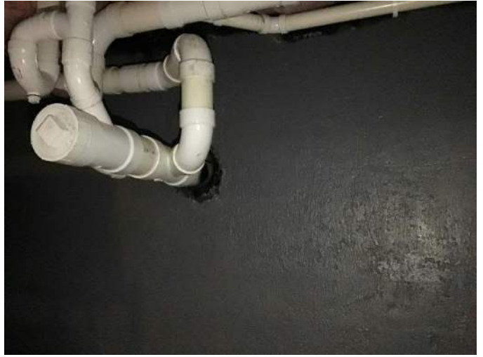
View of exposed PVC sewer lateral exiting into the concrete foundation to the backyard facing Southwest.
