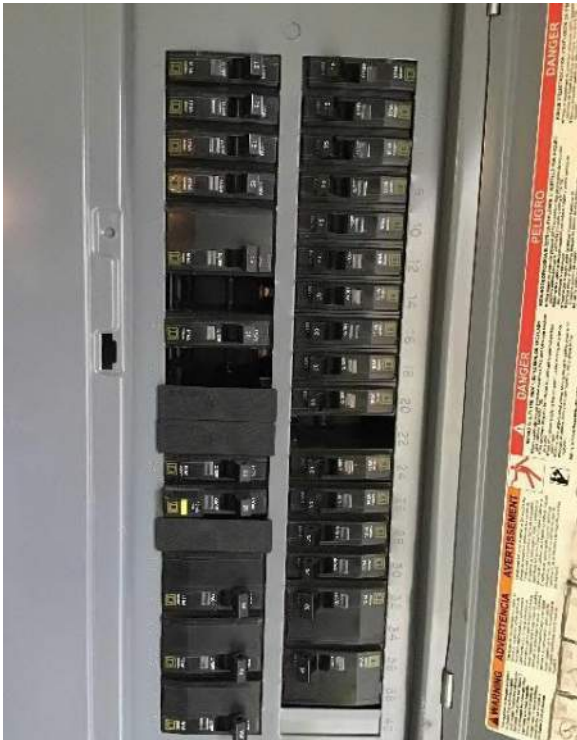
View of the breaker box circuit breakers.
