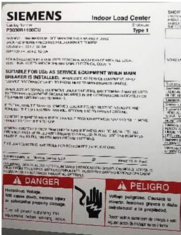
View of breaker box #1 model information and specifications.
