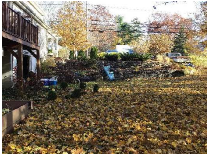
View of retaining wall and proposed sewer service pathway to the road, facing Northeast.
