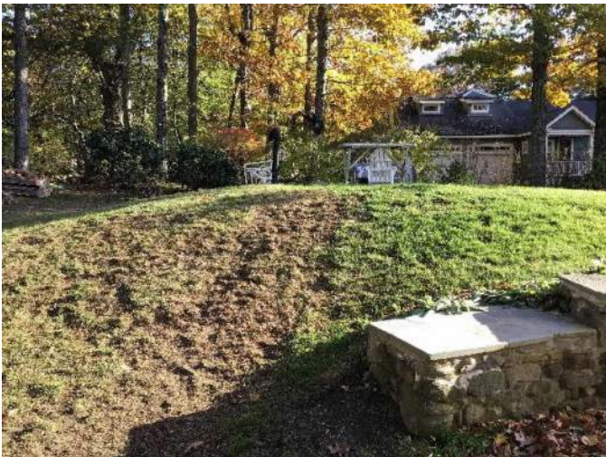
View of the leach field standing from the approximate location of the existing septic tank facing Southeast.
