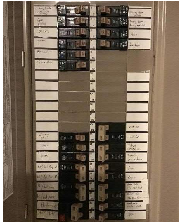
View of 200A breaker box #2 (Eaton) circuit breakers and schedule adjacent to breaker switches.
