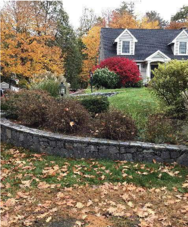
View of 241 Walker Bungalow Road and small retaining wall from the road facing Northeast.
