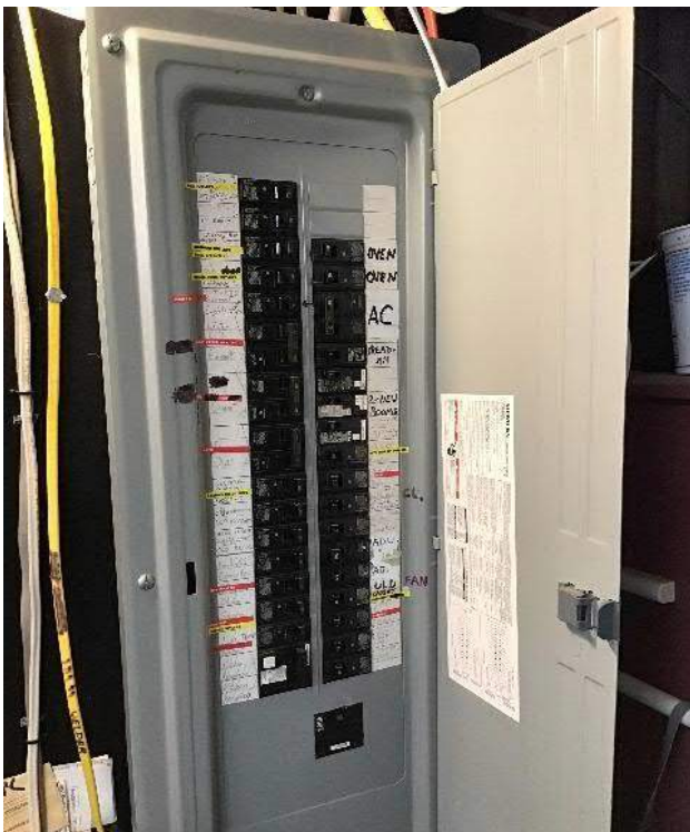
View of the breaker box with the panel front cover open.
