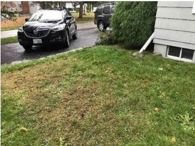
View of the septic tank and approximate location of the sewer lateral underneath the large shrub facing South
