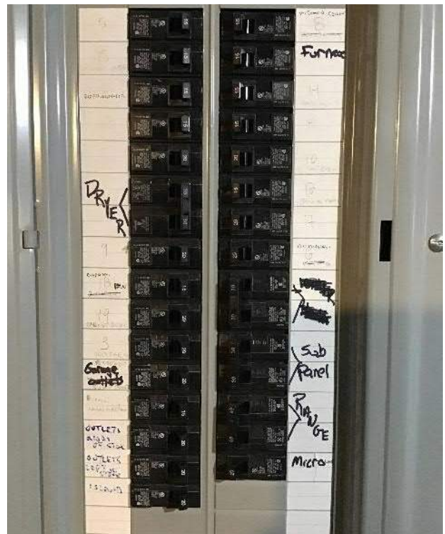
View of breaker box circuit breakers and schedule adjacent to the breaker switches.
