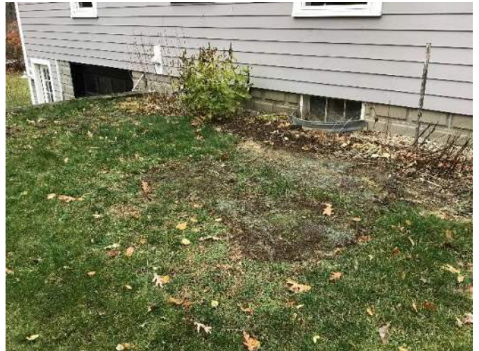
View of buried septic tank located next to the retaining wall with the leach field in the forefront, facing East.
