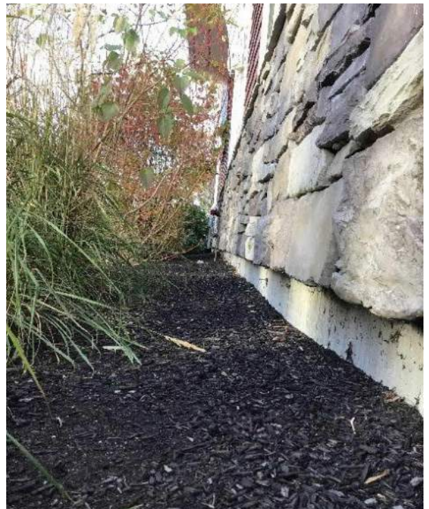
View of West exterior foundation and location of the sewer lateral exiting the foundation towards Sagamore Ave. facing North.
