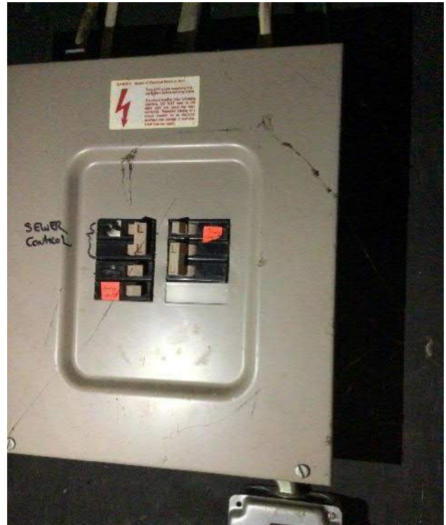
View of breaker box #2 and surrounding wall space facing Northeast.
