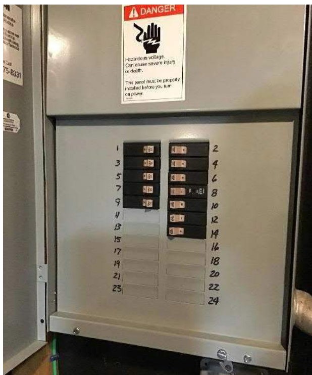
View of breaker box #2 (Eaton) circuit breakers adjacent to breaker box #1 facing Southwest.
