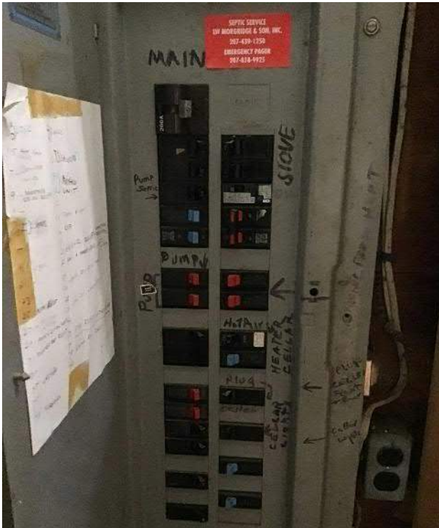
View of the breaker panel and surrounding wall space facing Northwest.
