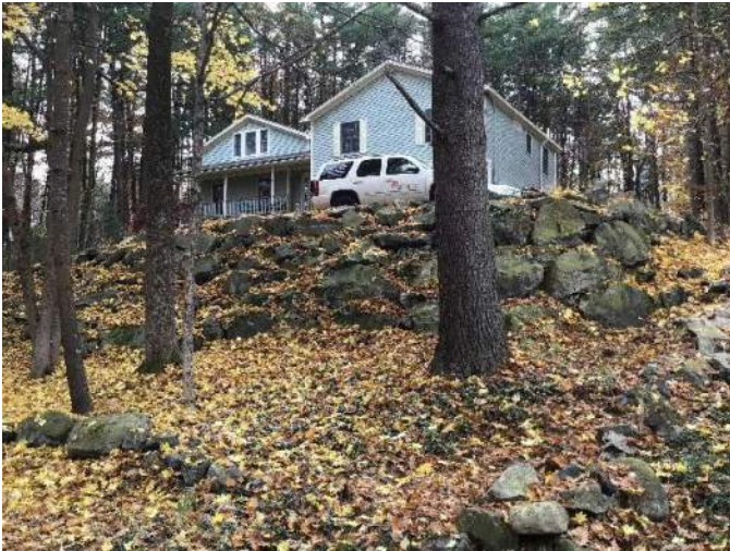
View of 40 Walker Bungalow Road and large retaining wall around the driveway from the road, facing Southwest.
