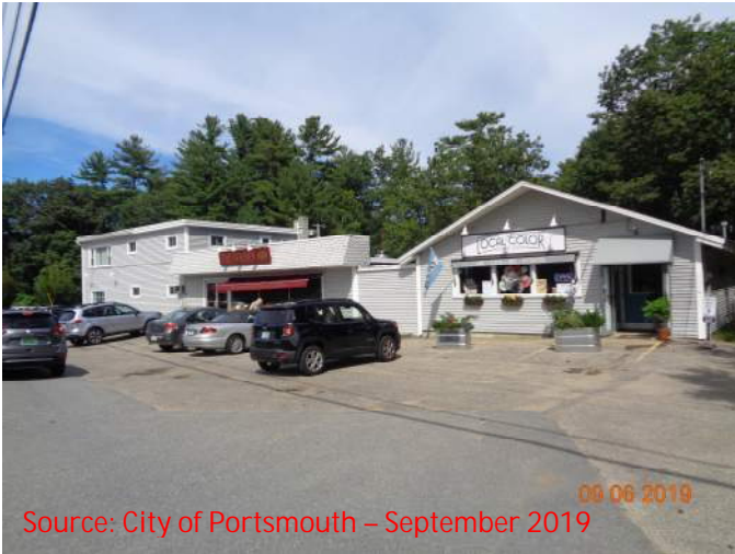
View of 960 Sagamore Avenue from the road facing Northeast.
