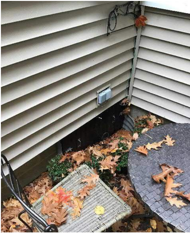
View of crawlspace access located next to the brick patio facing North.
