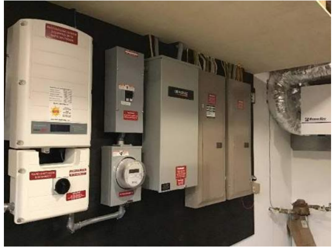
View of breaker boxes (#1 on left) and solar power electrical system facing South.
