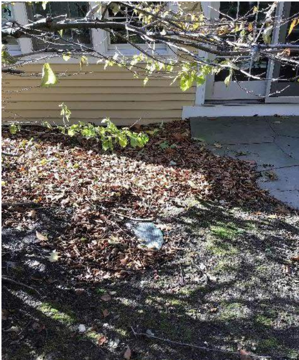
View of manhole cover for septic tank access located under a tree in the back yard facing Southwest.
