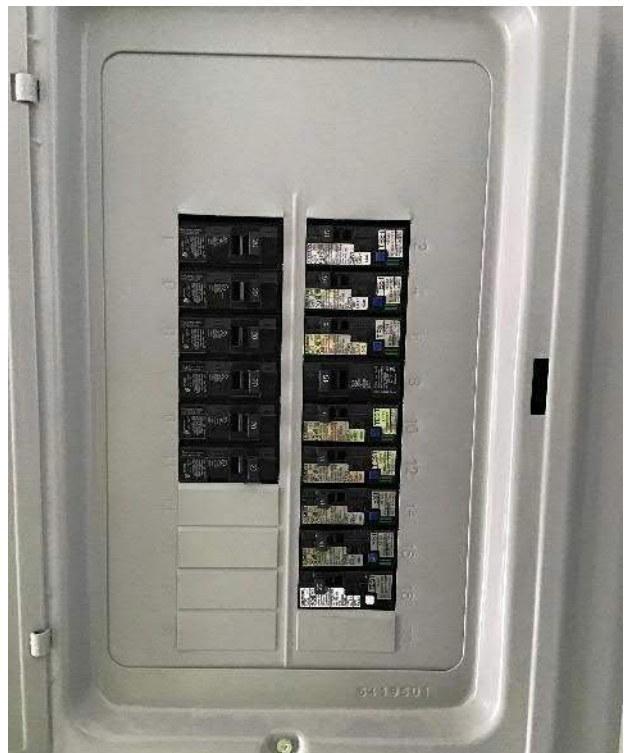
View of breaker box #2 (Siemens) circuit breakers.
