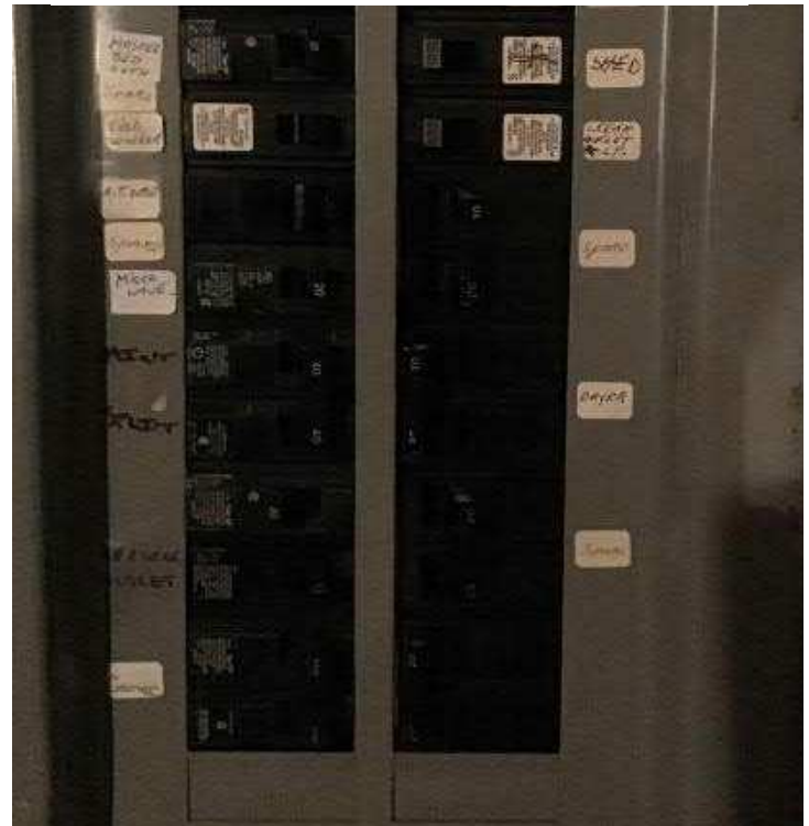
Continued view of breaker box circuit breakers and some schedule labels adjacent to the breaker switches.
