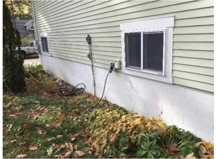
Exterior view of the exterior garage wall and location of sewer lateral exiting the foundation facing West.
