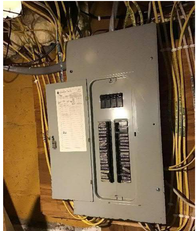
View of breaker box #1 and surrounding wall space facing North.
