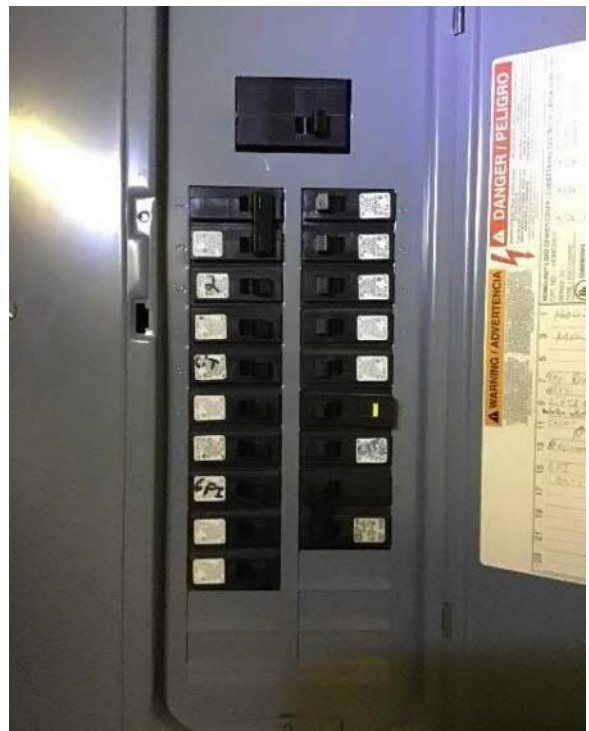
View of breaker box #2 (Homeline) circuit breakers.
