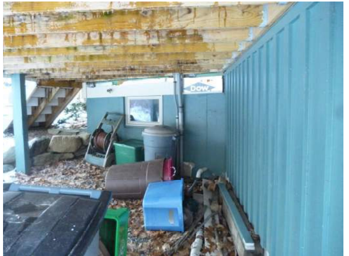
View underneath the raised wooden porch facing Southwest.
