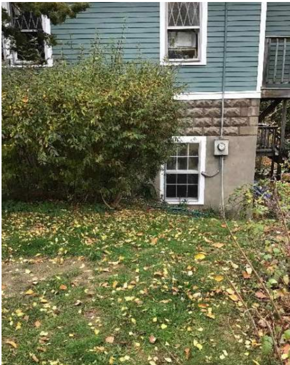
Exterior view of sewer lateral location facing Northeast.
