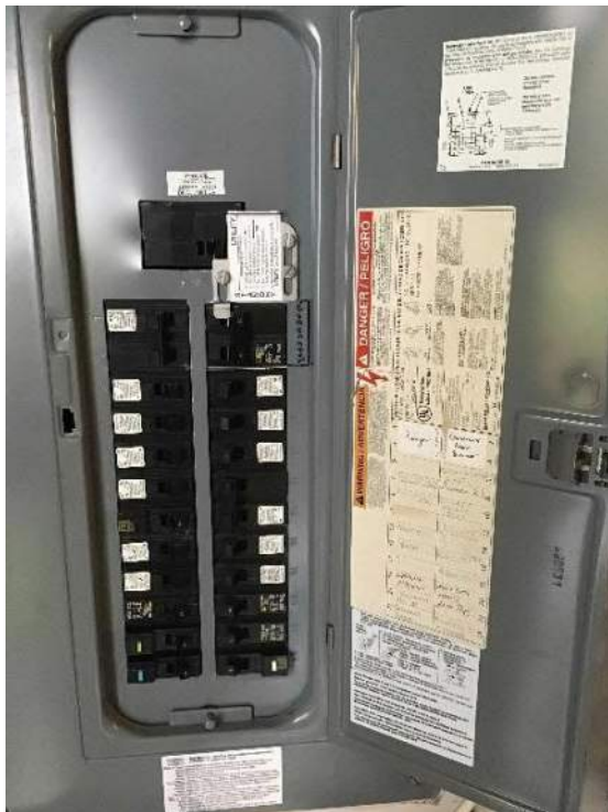
View of 100A breaker box open located on the Southeast wall of the garage facing Southeast.
