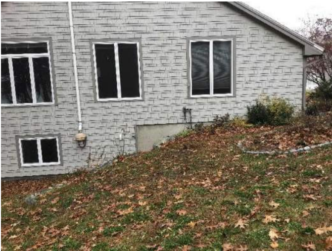
View of the approximate location of the sewer lateral and septic tank, facing East.
