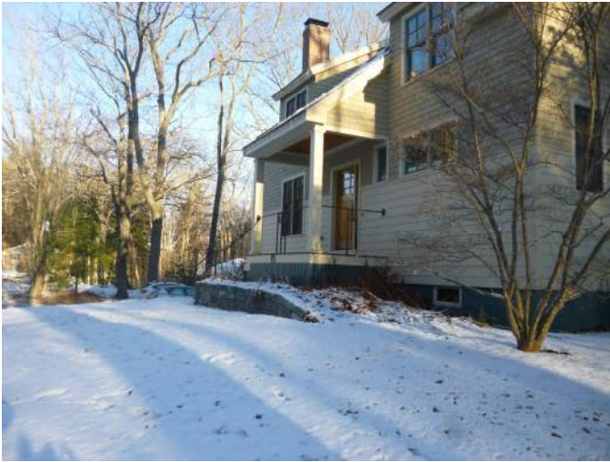
View of 93 Walker Bungalow Road and approximate location of the septic tank facing North.
