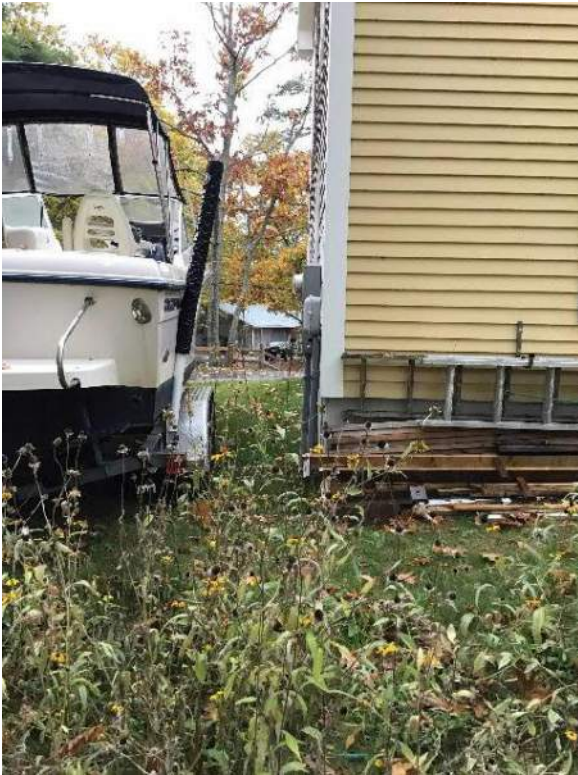
Exterior view of breaker box location on the garage wall facing Southwest
