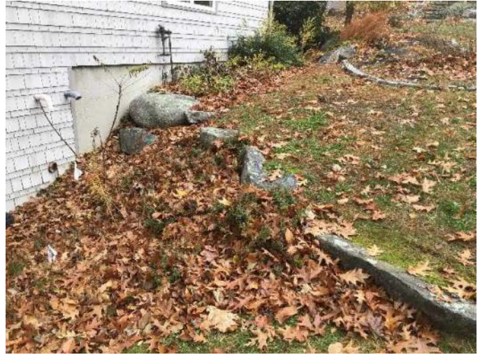
View of a small retaining wall near the approximate location of the buried sewer lateral facing North.
